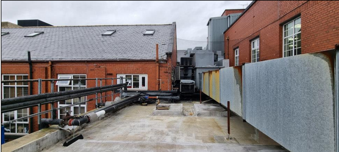
Plate 9: Elsewhere there were areas of flat roof with external plant; these areas offered no roosting potential.
