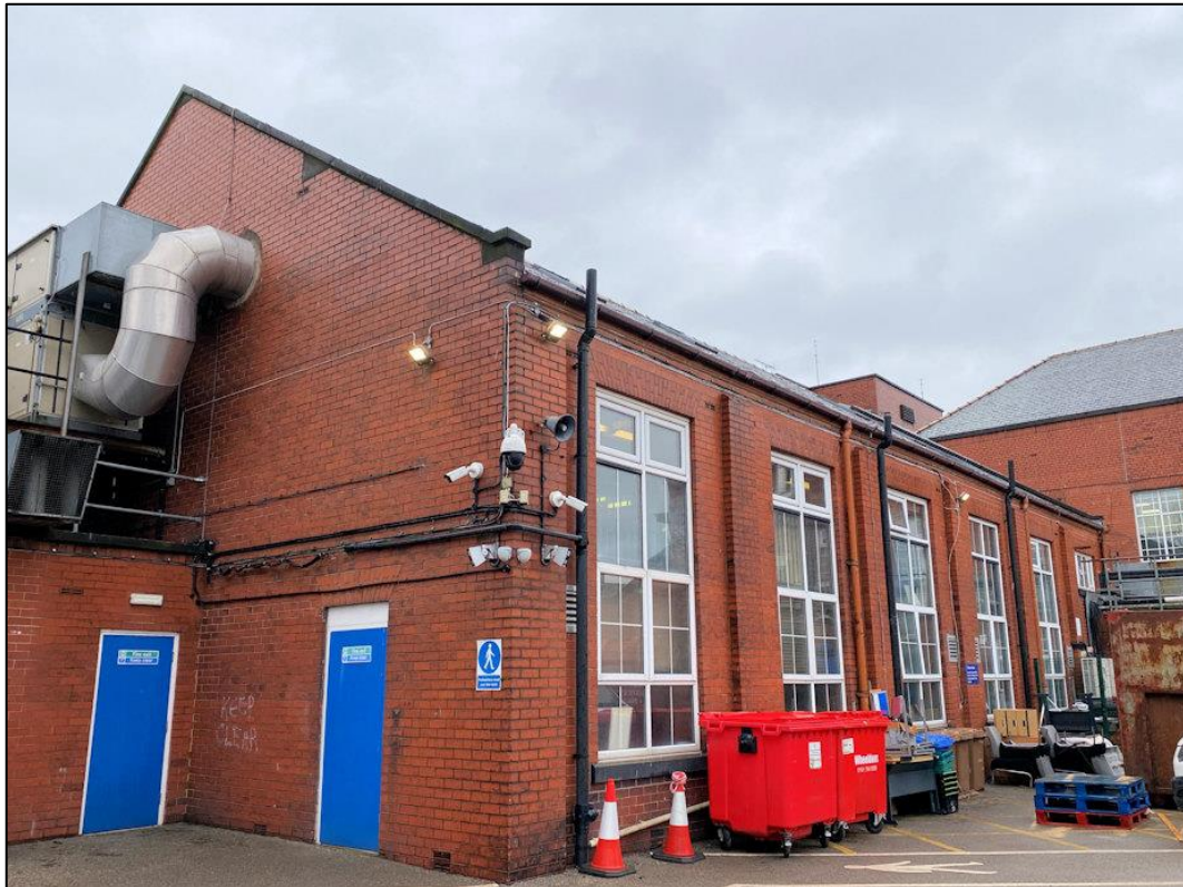
Plate 2: General view of the target building from the South.
