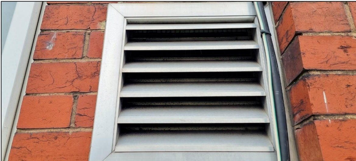
Plate 16: Vents had internal mesh preventing access for bats to the internal spaces.
