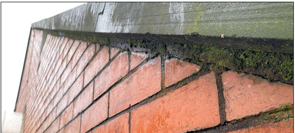
Plate 8: The mortar beneath the coping stones was generally intact and offered no roosting opportunities.
