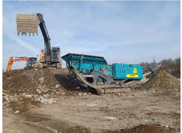
18.02.25 – Crushing of demo rubble
