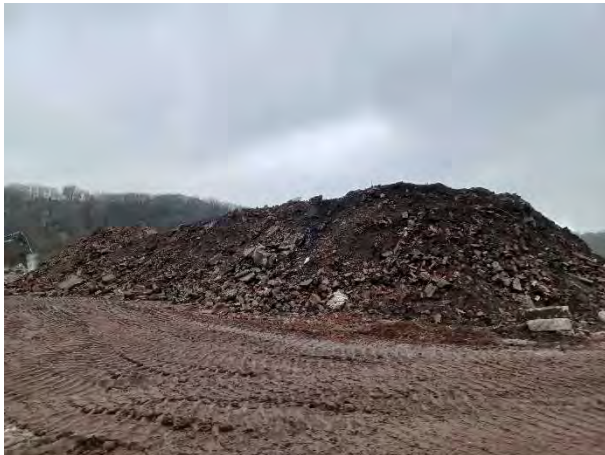
11.02.25 – Stockpiled demolition rubble of brick and concrete
