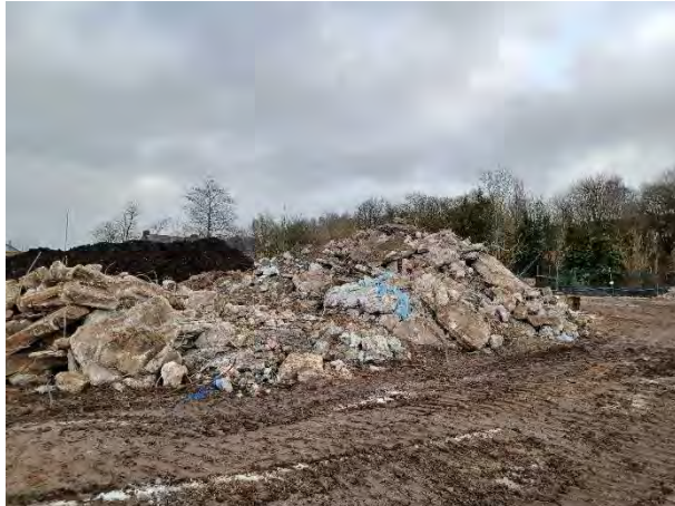
03.02.25 – Stockpiled recovered concrete awaiting processing
