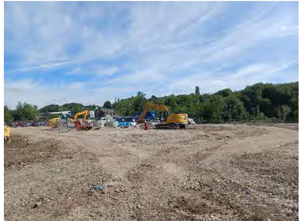
10.07.25 – Completed levels looking northeast
