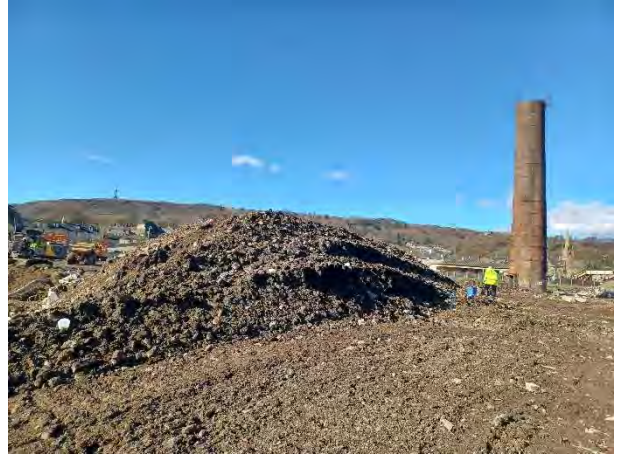
27.02.25 – Crushed demo rubble
