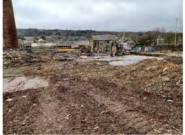
28.01.25 – One building remaining in the northwest within area where URL are locating services which enter the Site
