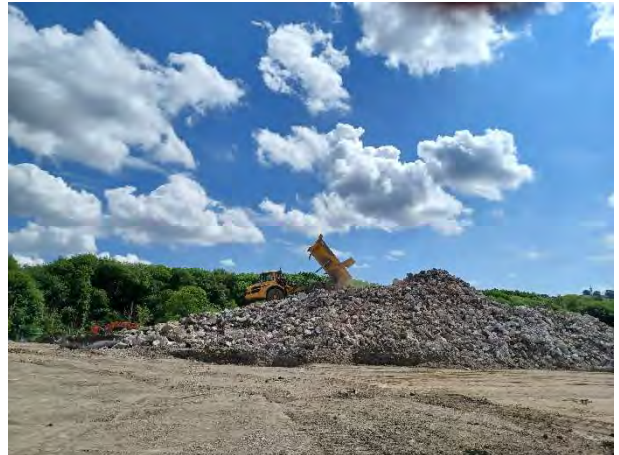
20.05.25 – Movement of material into stockpile
