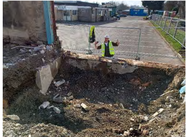
24.03.25 – Investigating southern wall footings
