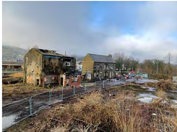
15.01.25 – Former mill buildings
