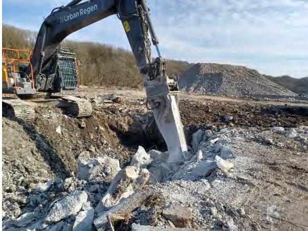
19.03.25 – Machine breaking out concrete
