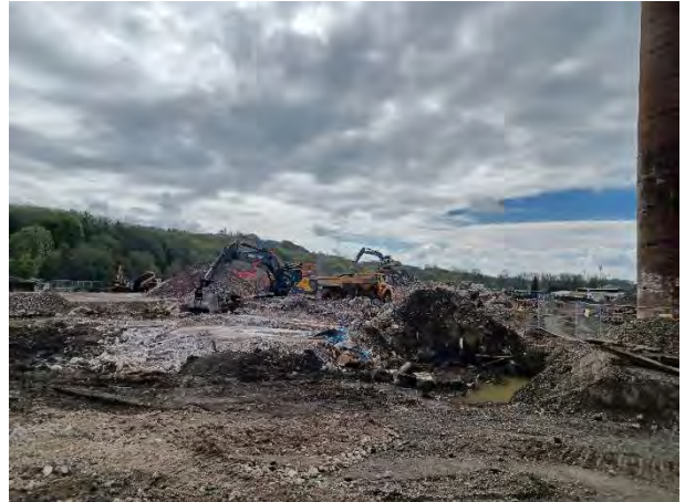
15.04.25 – Material movements across site
