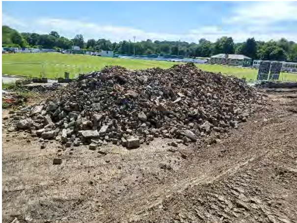
18.06.25 – Recovered demolition rubble ready for crushing
