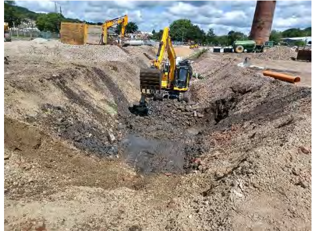
03.07.25 – Culvert works in southwest
