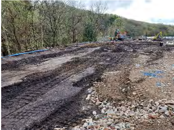
15.04.25 – Regrading along east boundary
