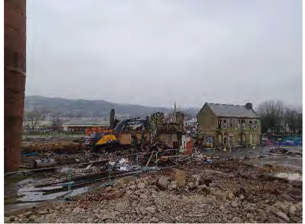
23.01.25 - Demolition of former mill buildings in progress
