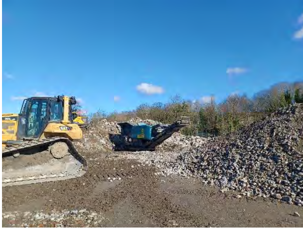
27.02.25 – Crusher crushing concrete
