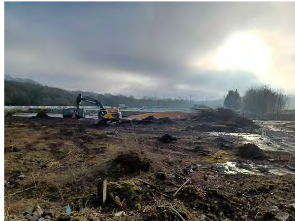
15.01.25 – View south across Site
