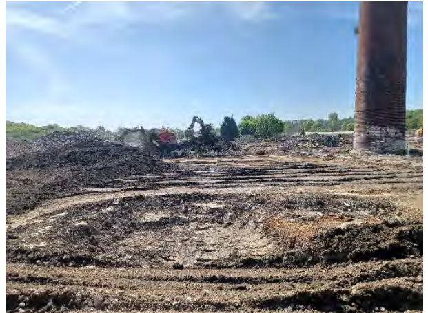
30.04.25 – Regraded area in centre
