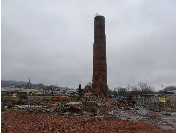
23.01.25 – Demolition of former mill buildings in progress
