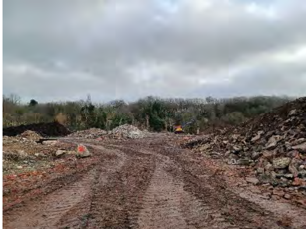
03.02.25 – View east following demolition
