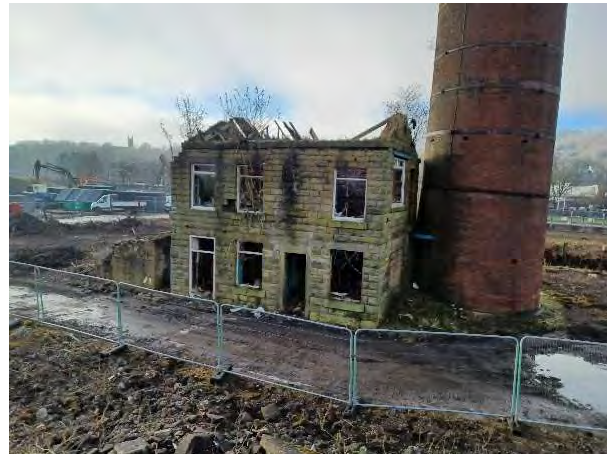
15.01.25 – Former mill building and chimney
