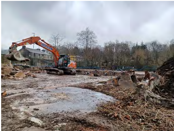
11.02.25 – Machine moving oversized concrete
