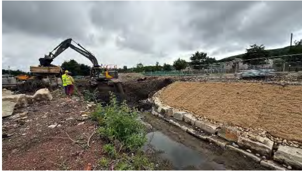
26.06.25 – Preparing for placement of culvert
