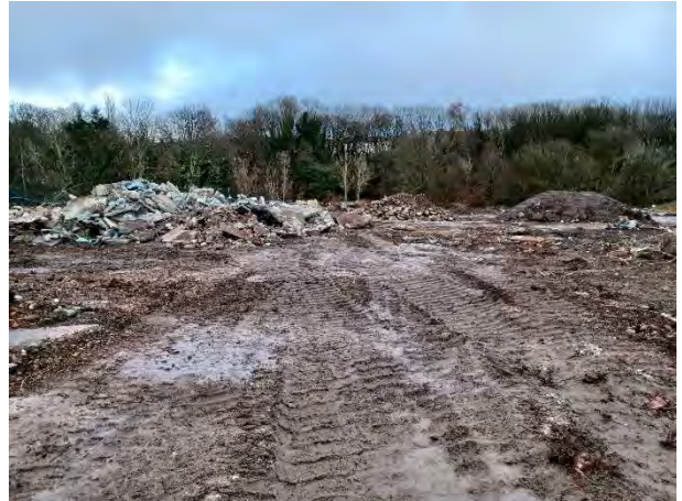
28.01.25 – Eastern view following clearance of scrub vegetation
