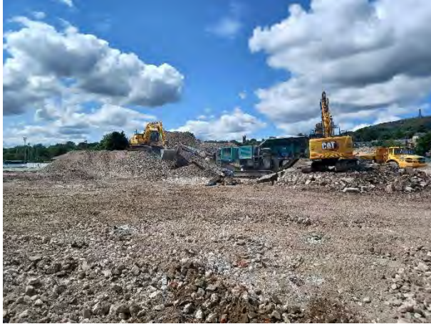
03.07.25 – Crushing in the south
