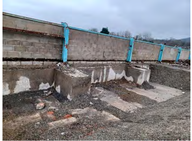
11.02.25 – Retaining wall on south boundary
