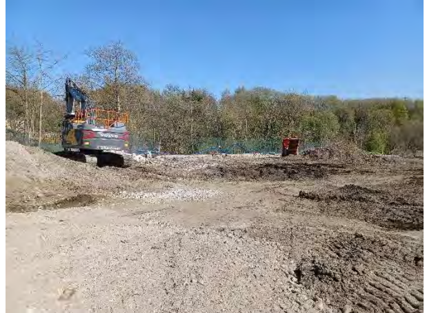
10.04.25-Regrading in northeast
