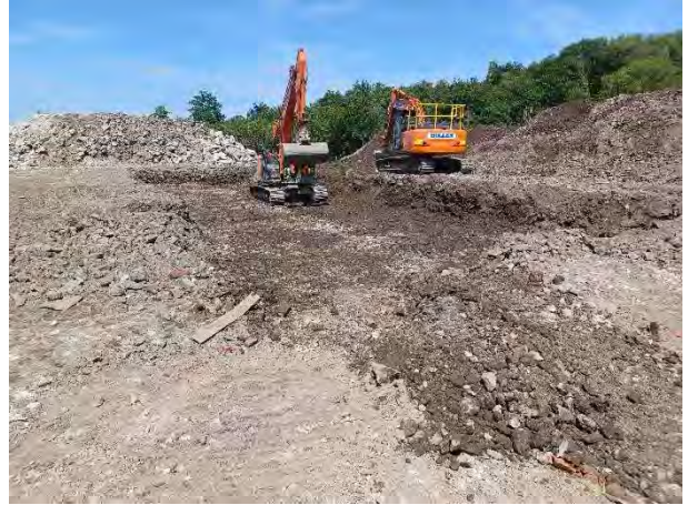
18.06.25 – Regrading for replacement of crush
