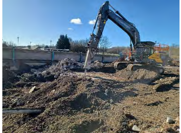
27.02.25 – URL breaking out concrete in south
