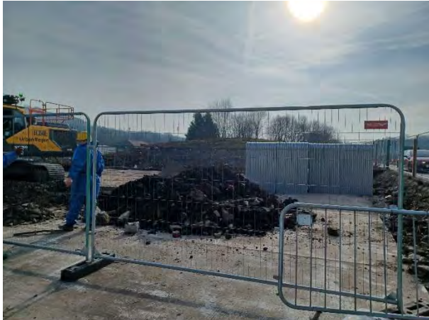
18.02.25 – Asbestos stockpile being handpicked by train URL operatives
