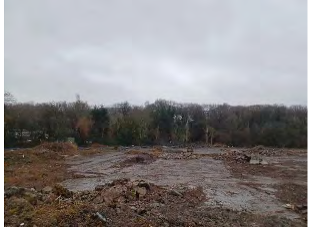
23.01.25 – View east across Site
