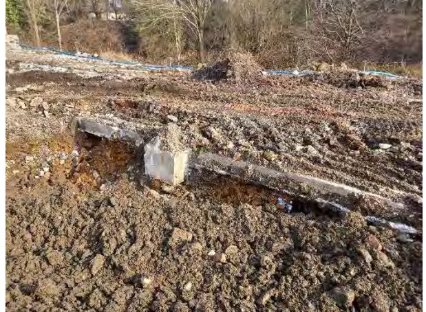
18.02.25 – Slab in west of Site
