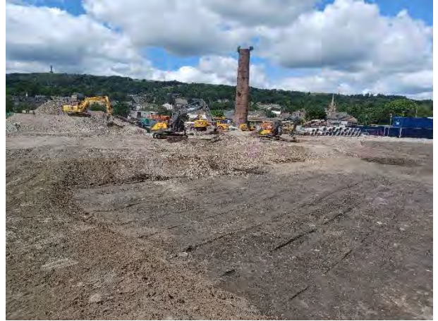
03.07.25 – Completed levels in east
