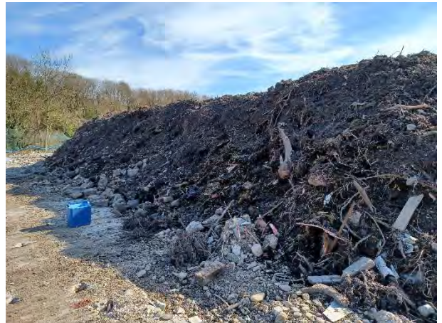
05.03.25 – Stockpile of organic soils recovered from site pending testing to establish potential for reuse
