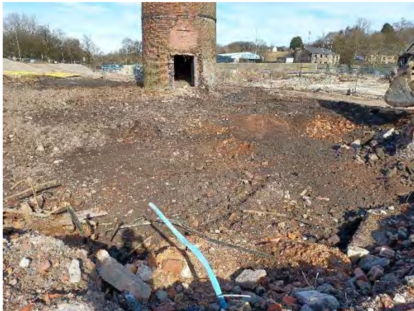
05.03.25 – Turnover of made ground taking place to the south of the chimney (former boiler house)
