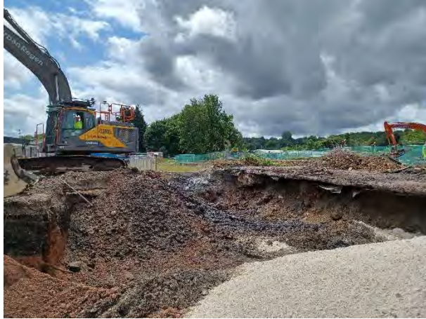
06.06.25 – Slab removal in southwest
