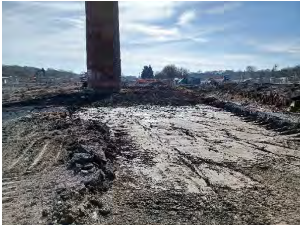
05.03.25 – Turnover soils completed to the north of chimney
