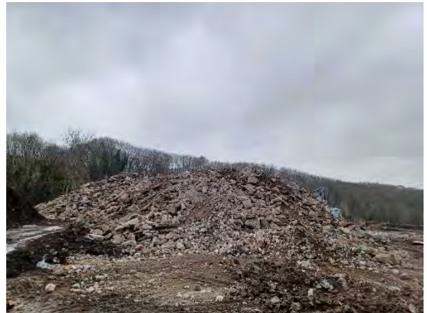
11.02.25 – Stockpiled oversize awaiting processing
