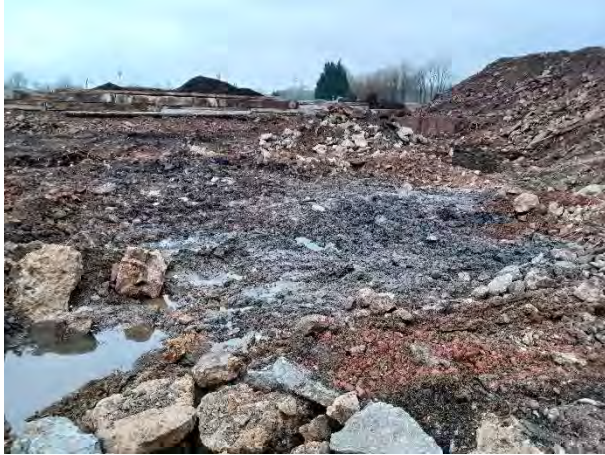
11.02.25 – Area of very soft silty clay where old piles were removed
