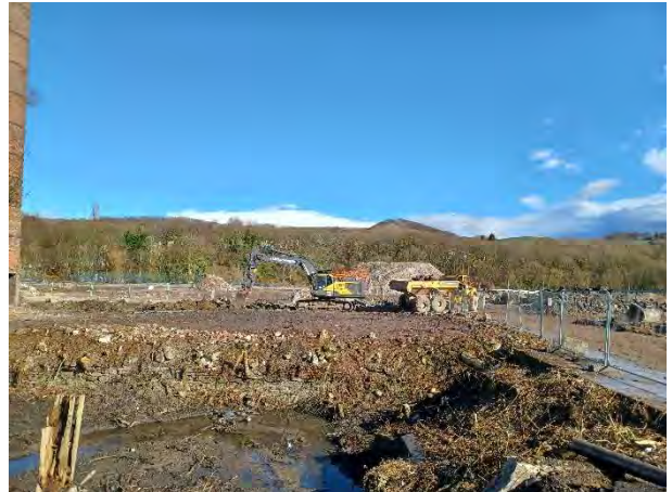
11.03.25 – Machine removing road near chimney
