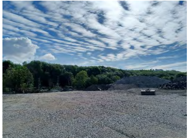
07.05.25 – Regraded north / centre area
