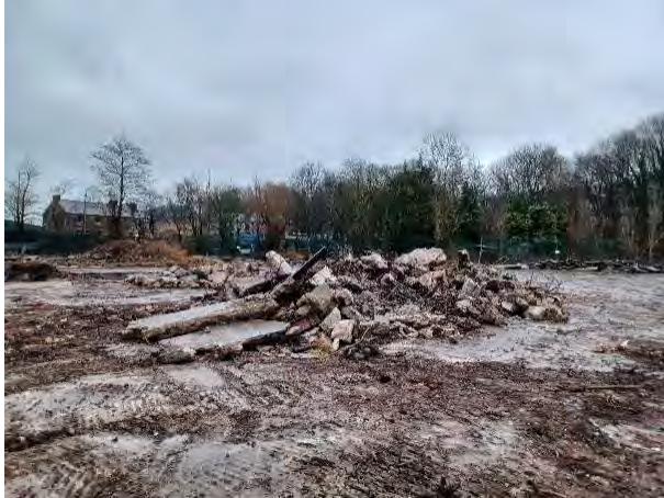
23.01.25 – Stockpiled recovered materials
