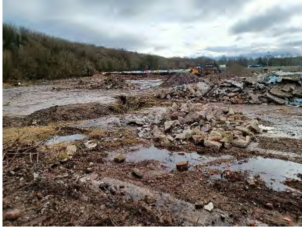
28.01.25 – Southeast view with previously broken out hardstanding stockpile awaiting processing
