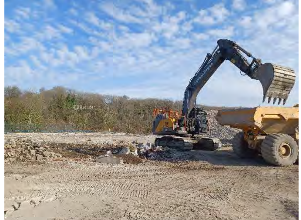
19.03.25 – Transferring of concrete
