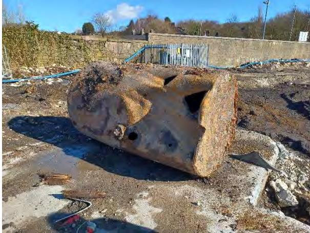
27.02.25 – Pulled tank from north boundary
