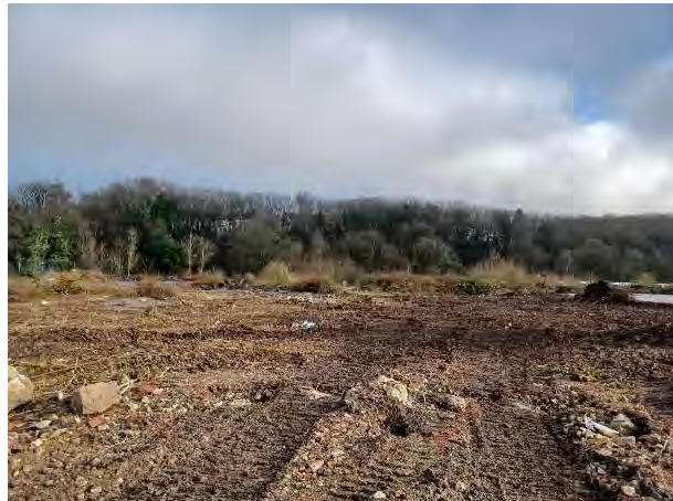
15.01.25 – View east across Site
