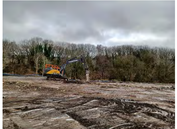
03.02.25 – Machine breaking out concrete in the east
