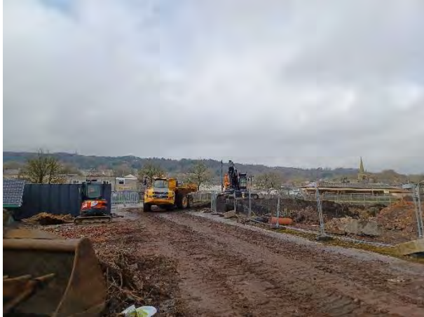
03.02.25 – Machine clearing northwest boundary of mounded soils
