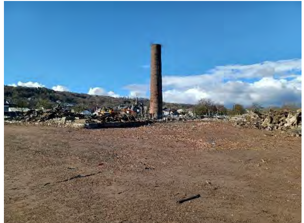
11.03.25 – Phase 1 completed turnover
