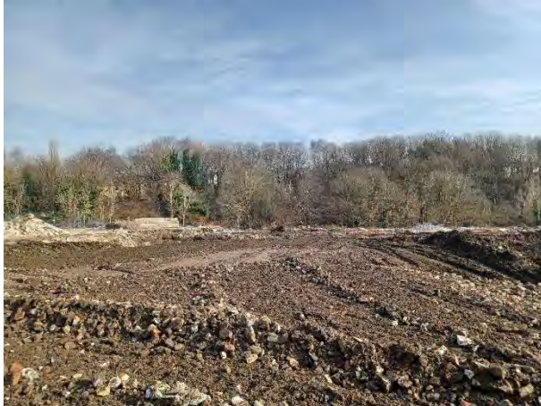
18.02.25 – Crushed demo rubble used to raise levels
