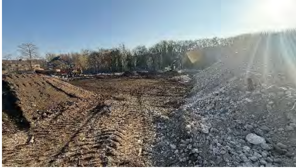
03.04.25-Machines regrading site in northeast
