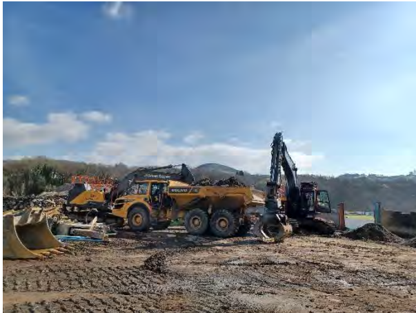
24.03.25 – Machines removing material from southern wall footings
