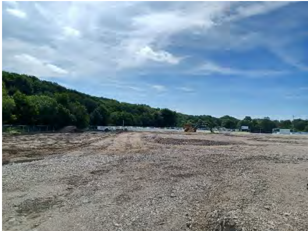
10.07.25 – Completed levels looking south
