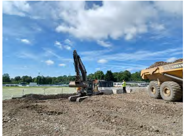
10.07.25 – Final area placing levels (southeast)
