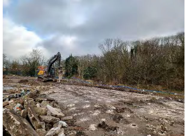
03.02.25 – Machine pecking concrete on west boundary
