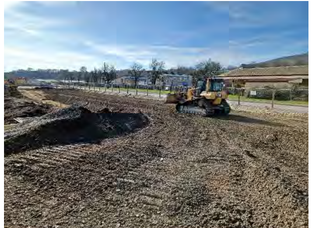
05.03.25 – Regrading site-won sub-base material in the northwest
