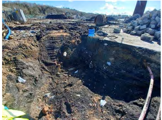
27.02.25 – Tank pull area
