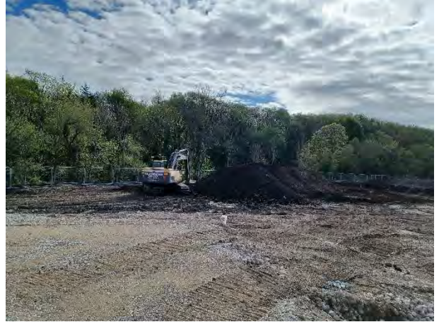
23.04.25 – Regrading in southeast corner
