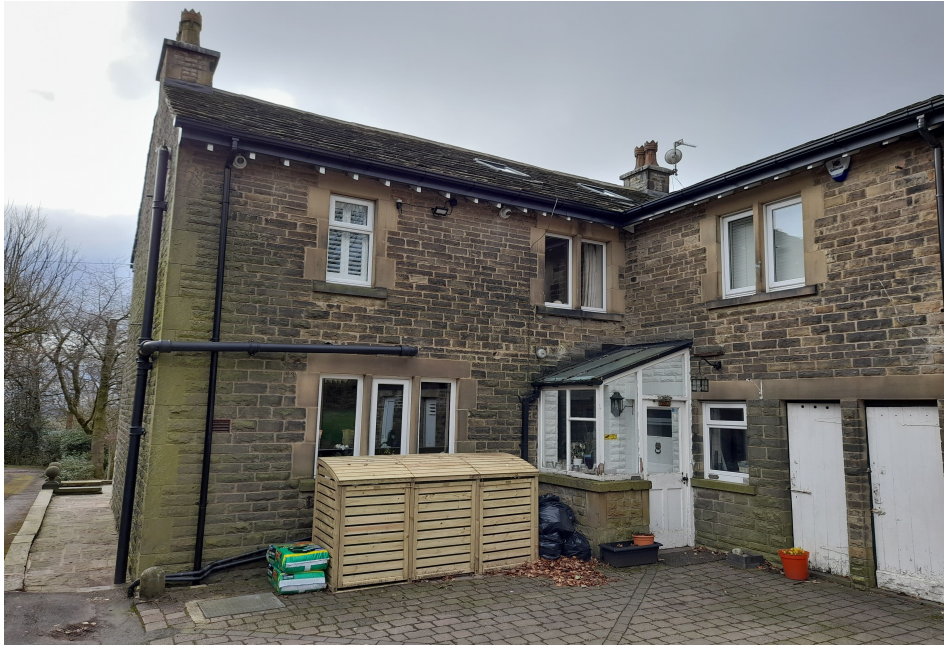
view of existing part northern elevation .
