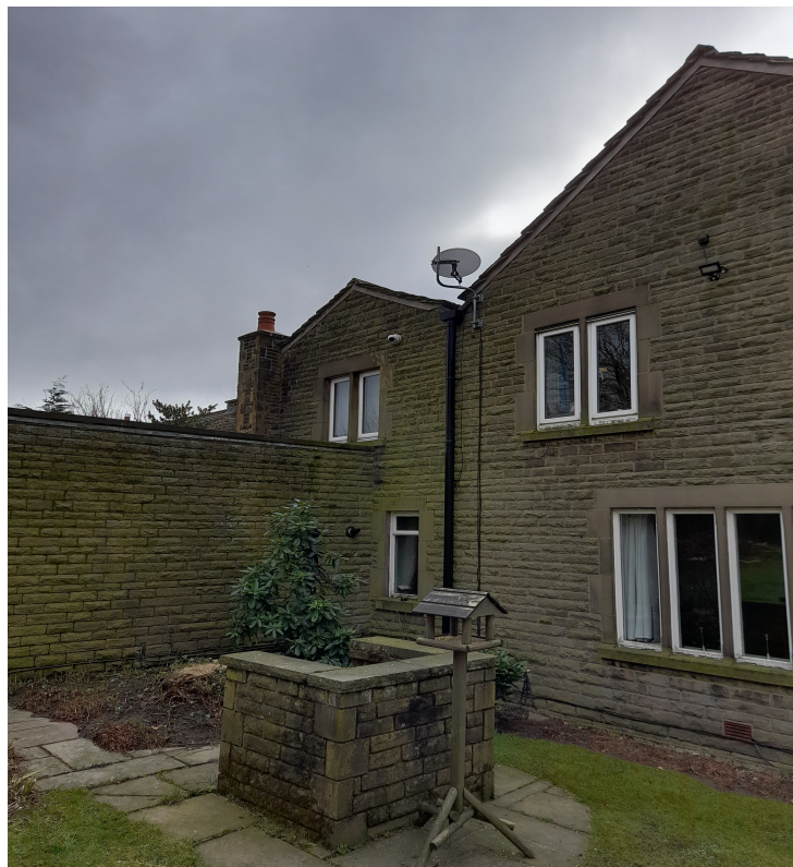
View of part northern elevation.
