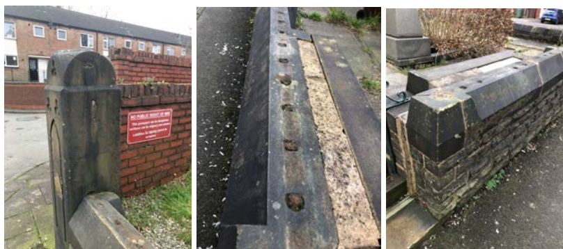
Image 02: Remnants of previously installed perimeter railings
