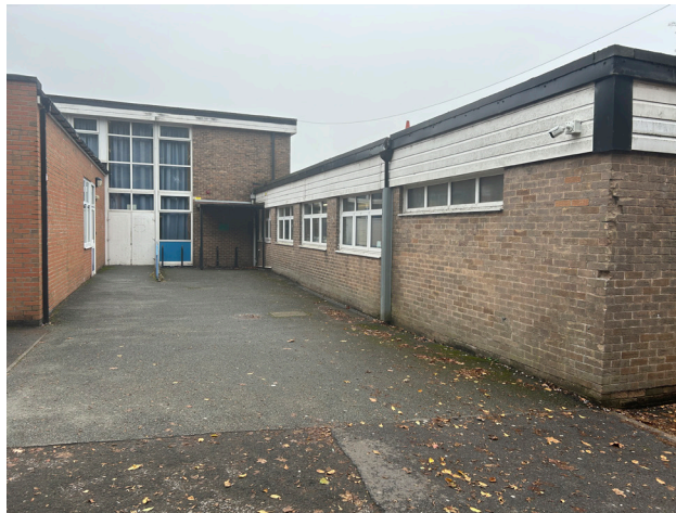
Rear of kitchen abutting main school hall.
