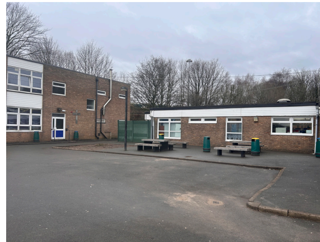
Adjacent 2-storey teaching block.
