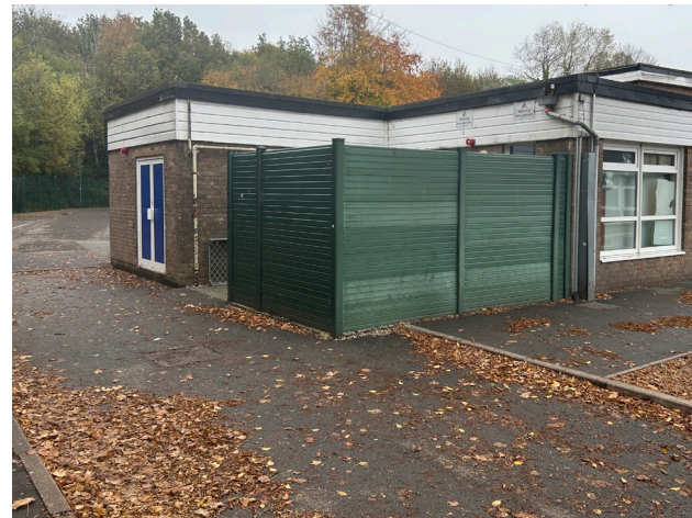
Store and bin enclosure to gable end of kitchen.
