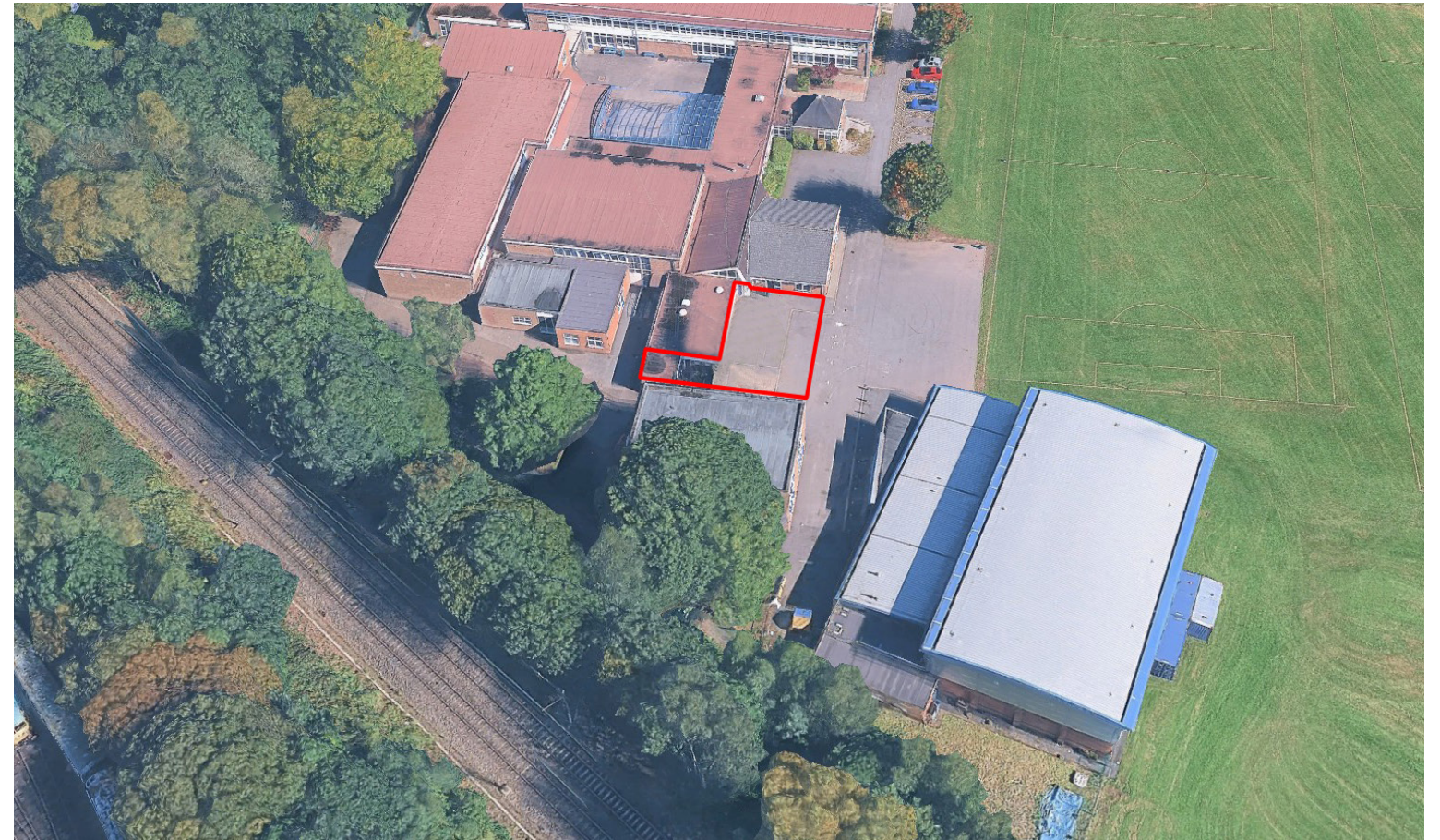
Aerial image of the school site showing massing of the school buildings and proposed development area..
