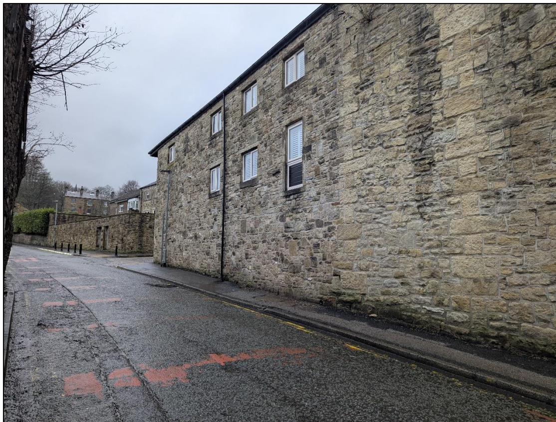
Plate 9: View north along Kay Brow showing rebuilt wall
