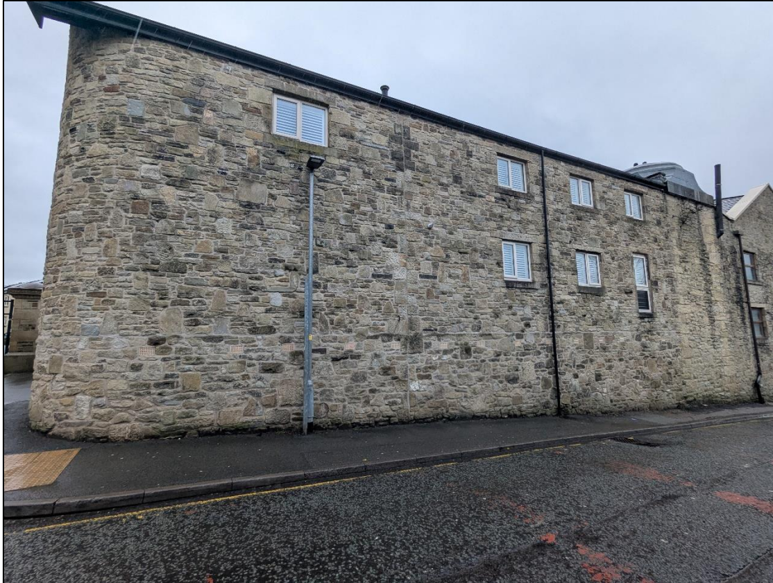
Plate 8: Southern rebuilt wall of gate house with remains of chimney to the far right
