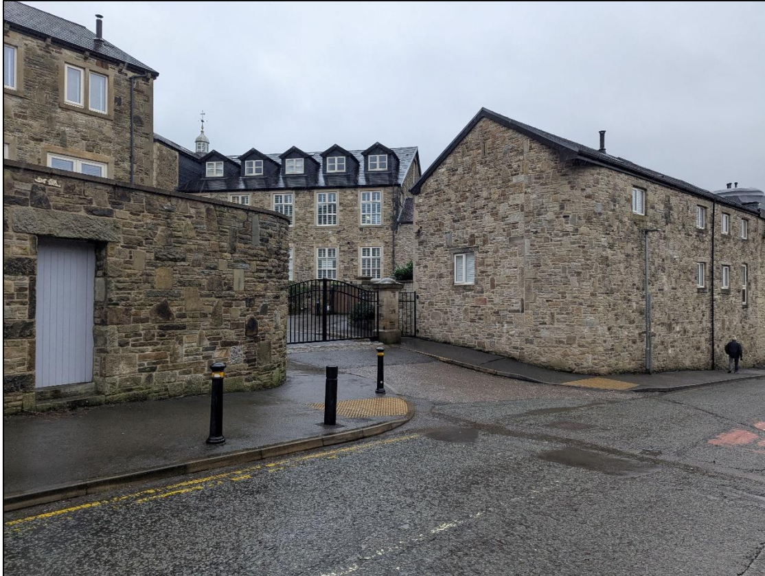
Plate 6: Entrance from Kay Brow and gate house to the right
