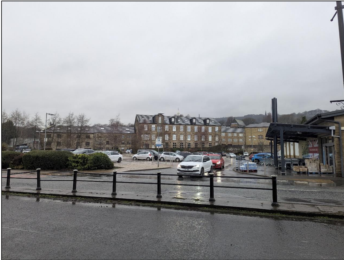
Plate 1: View of East elevation of Cobden Mill from Railway Street
