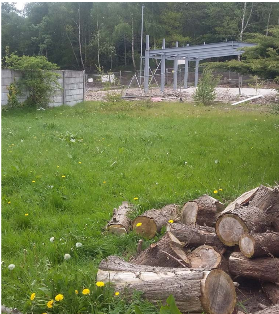
Photograph 1: View north west of the Site
