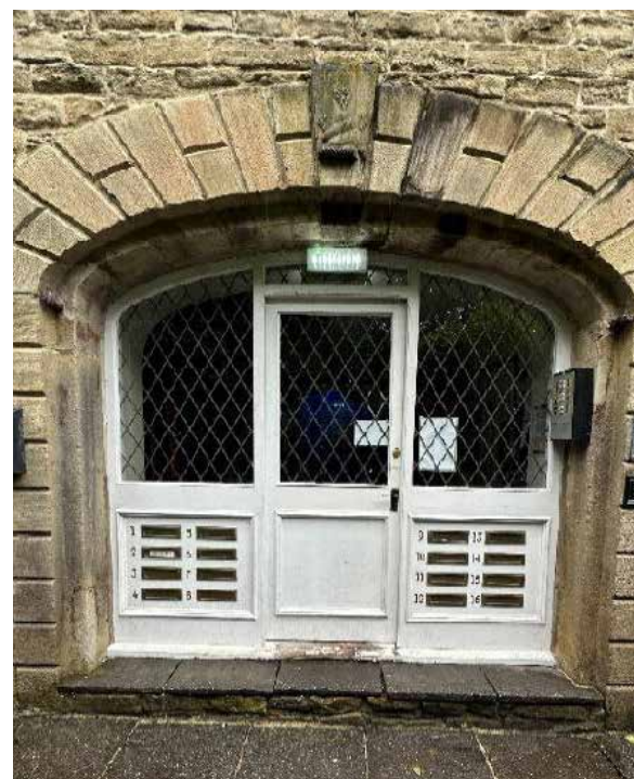
Existing Door Condition
