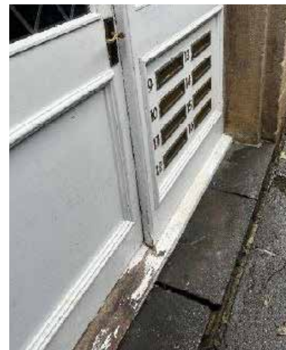
Existing Door Condition
