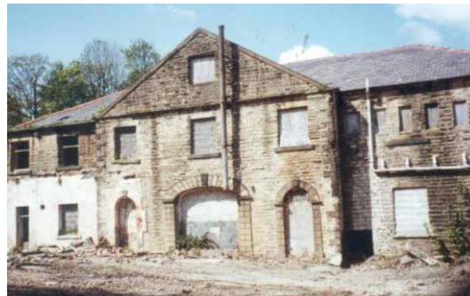
Barwood Lea Mill - Before Residential Development
