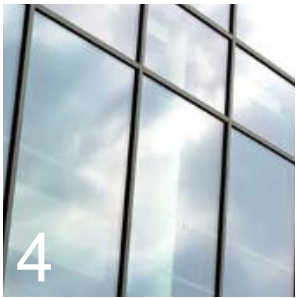
Dark grey parapet capping and window frames
