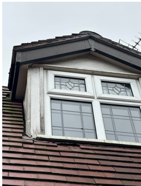
6 – Front tiles are in good condition. There are some small gaps around the dormer but there is lead flashings and felt behind. Fascias and soffits are all closed UPVC construction.
