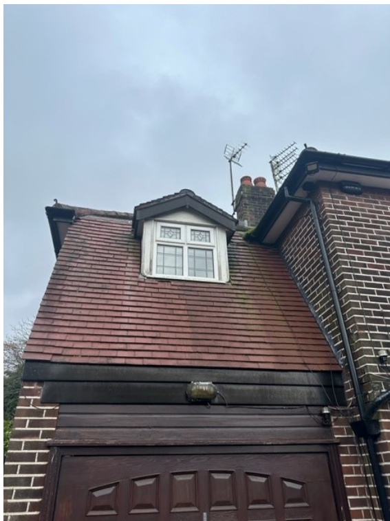
6 – Front tiles are in good condition. There are some small gaps around the dormer but there is lead flashings and felt behind. Fascias and soffits are all closed UPVC construction.
