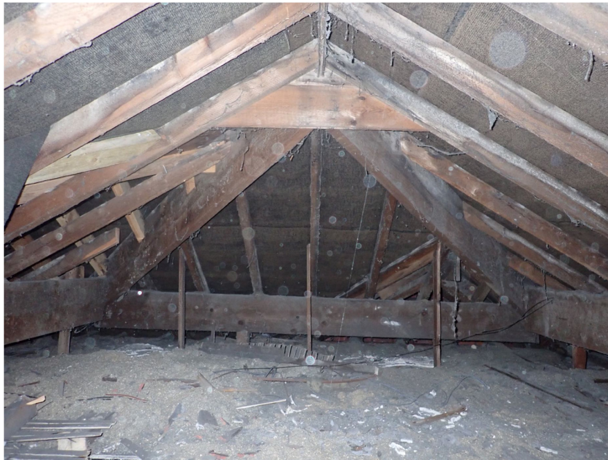
3.2a – Typical main roof void.
