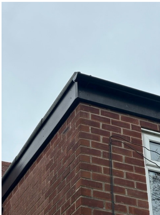
4– UPVC fascia boards and soffits at the eaves are fixed tightly against brickwork. UPVC windows are all in good condition and tightly fixed with silicone sealant.
