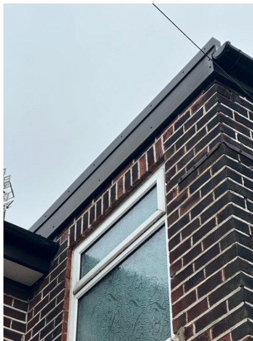
4– UPVC fascia boards and soffits at the eaves are fixed tightly against brickwork. UPVC windows are all in good condition and tightly fixed with silicone sealant.
