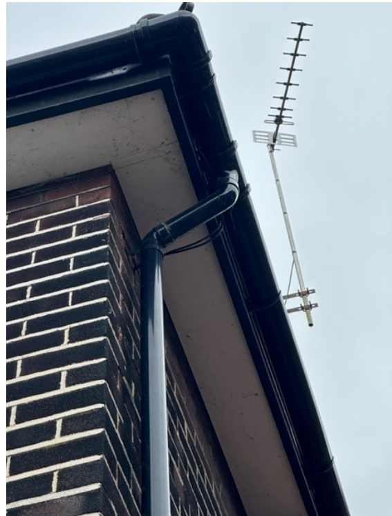
5 – Brickwork and mortar and boxed eaves are in good condition with no suitable gaps.
