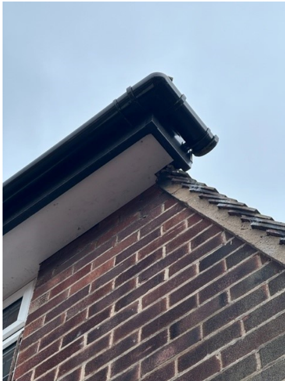
5 – Brickwork and mortar and boxed eaves are in good condition with no suitable gaps.
