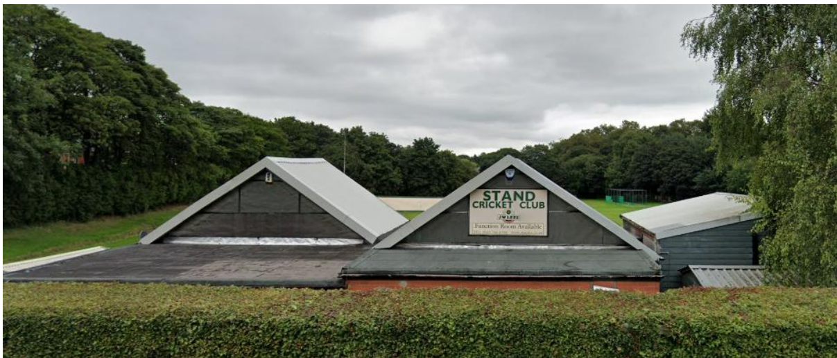
Figure 3 – site partially obscured
