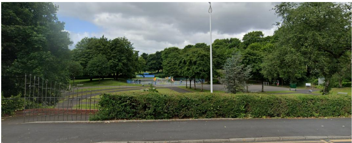
Figure 7 – View of site from Bury New Road
