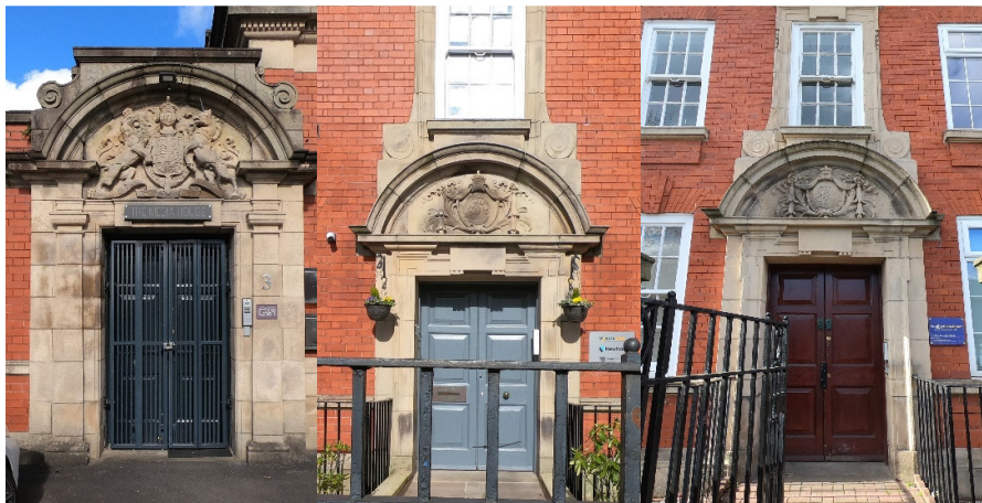
Original entrance surrounds with stone entablatures
