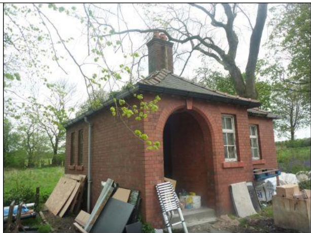
Photo 7: Southern and eastern elevation of Building 1
