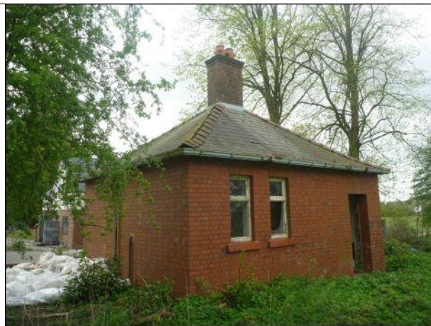
Photo 8: Northern and western elevation of Building 1
