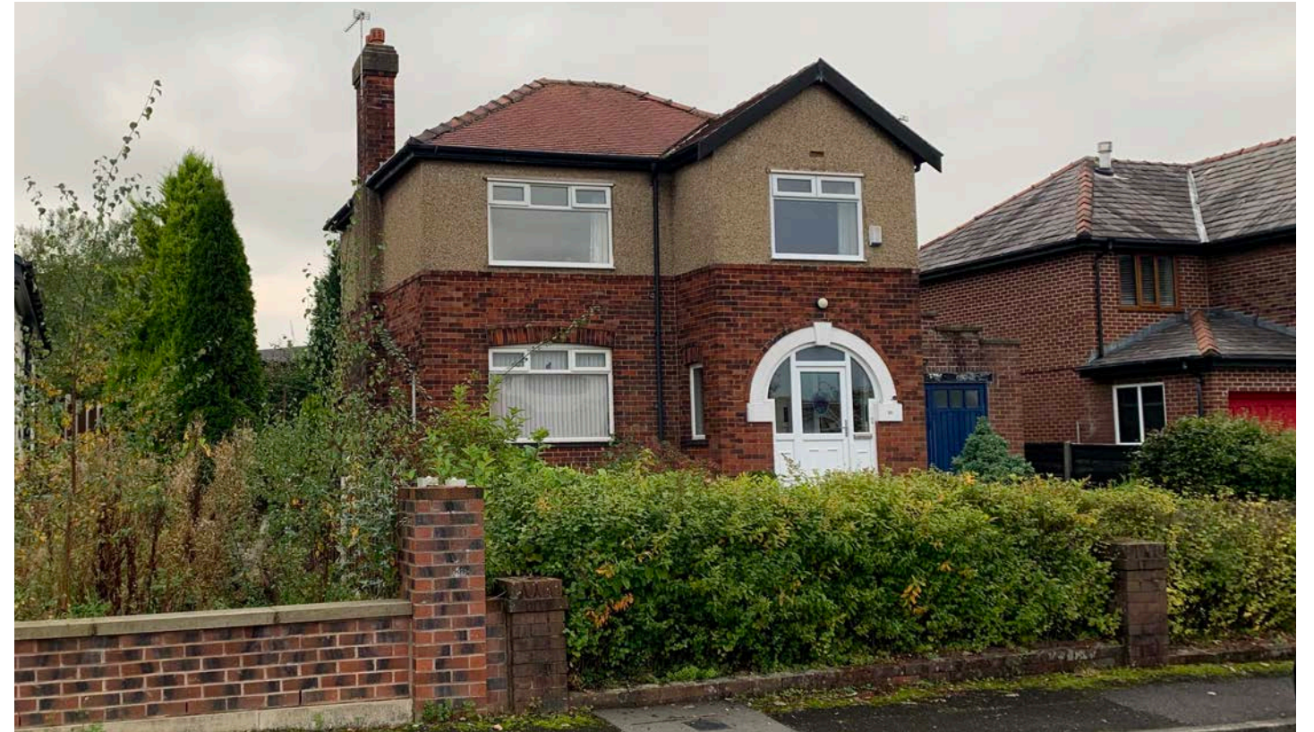
Above: Existing House - Front
