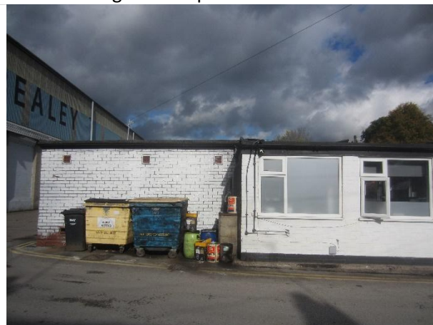
Photo 18: Western elevation of building B1
