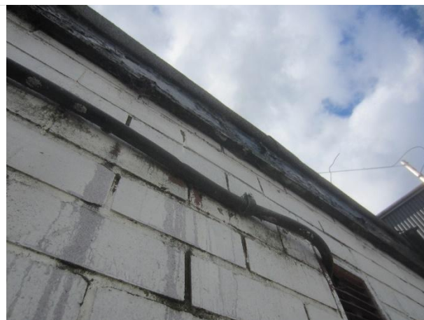
Photo 20: Example of brick elevation walls and fascia at building B1
