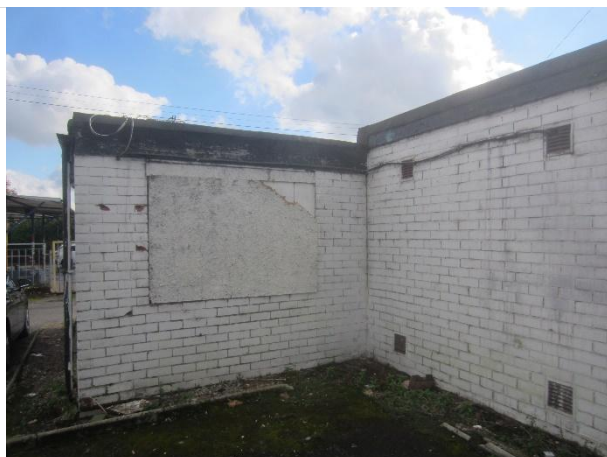
Photo 19: Northern and eastern elevations of building B1
