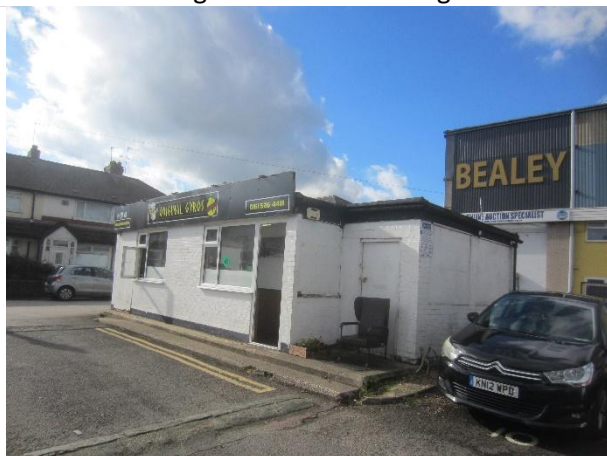
Photo 17: Southern elevation of building B1
