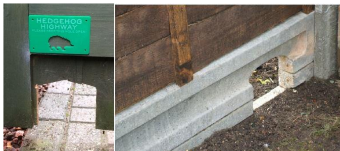
Insert 4: Showing wildlife access gap within fencing
