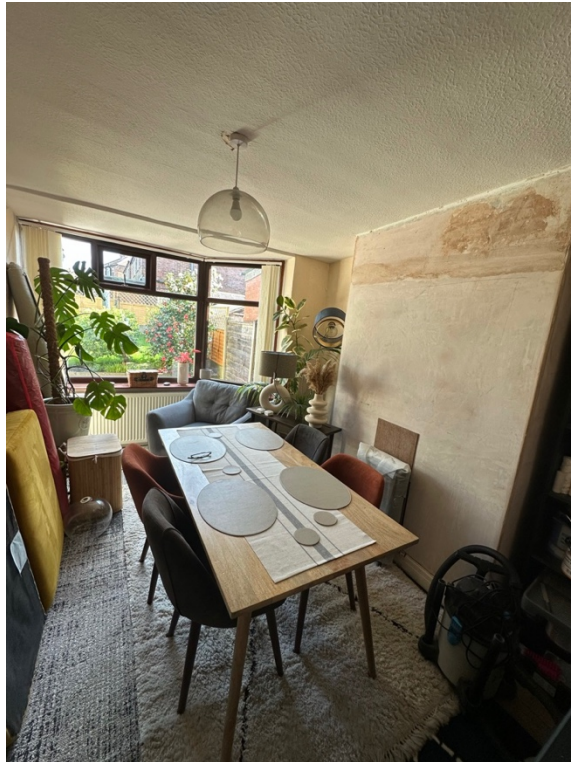
Figure 3 - Existing dining room which will become the new kitchen.
