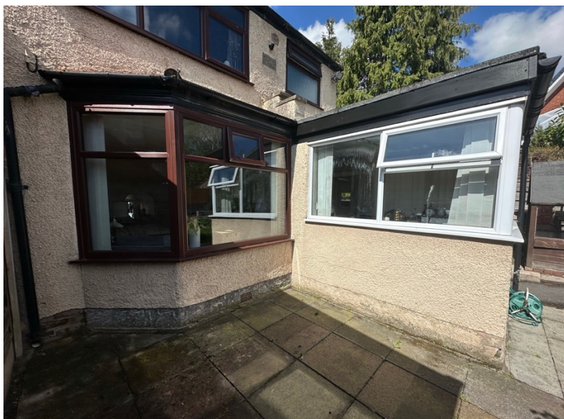
Figure 2 - Rear Bay window of existing dining room, and the courtyard space which would become part of new extension
