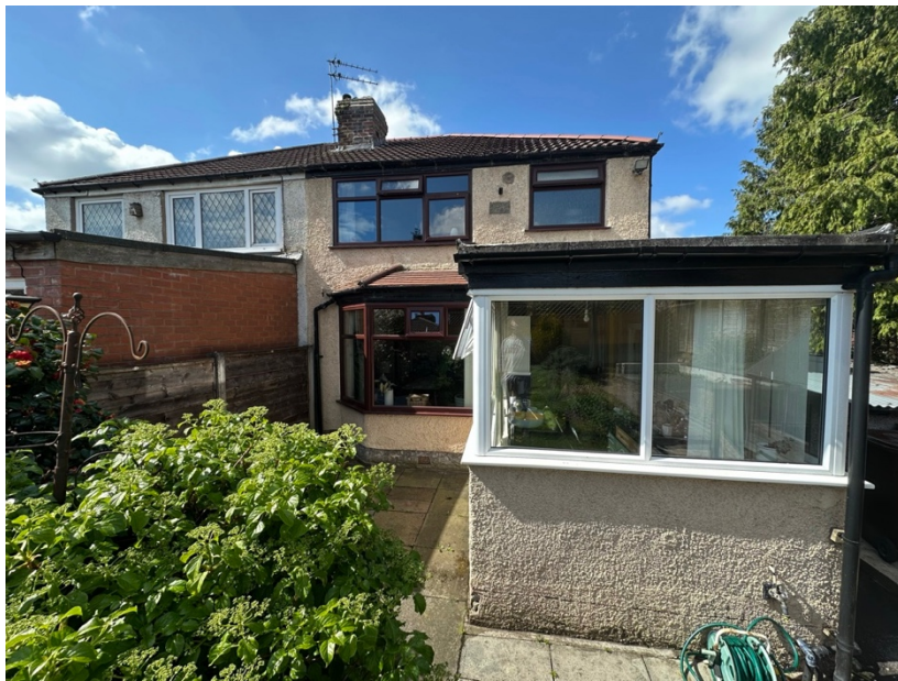
Figure 1 - Existing rear elevation showing single storey kitchen extension
