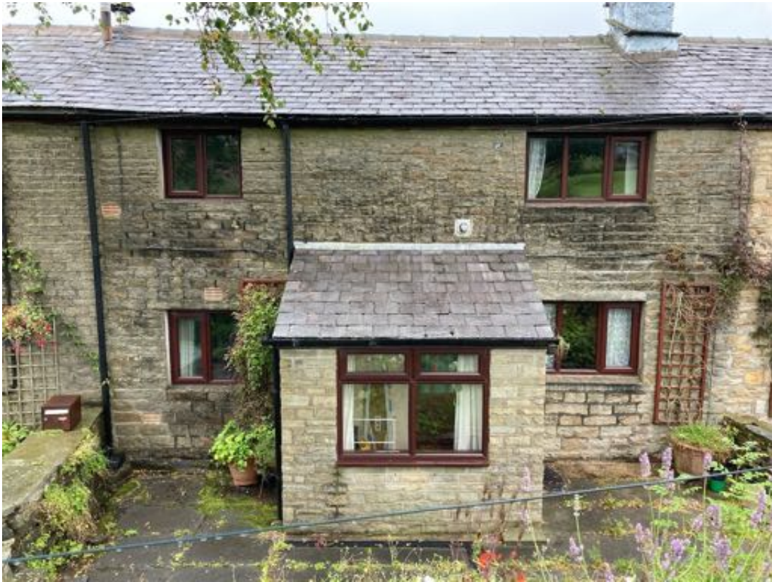
Figure 1: View of the front elevation of 322 Turton Road.
