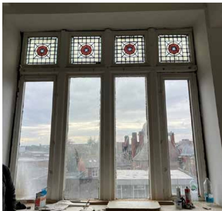
Image: Original windows to upper floor.
