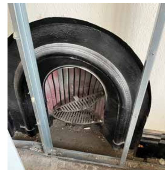
Image: Example of remaining fireplace to upper floor.
