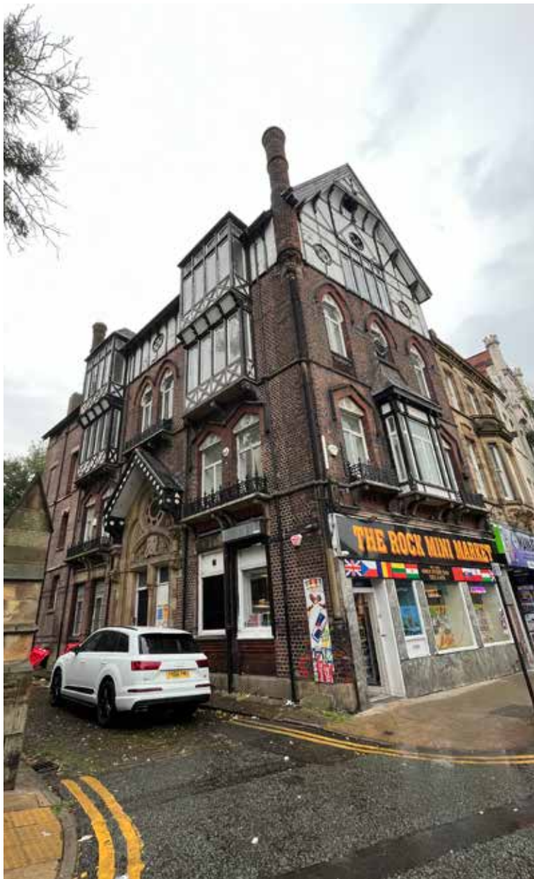
Image: Union Buildings, primary elevations.
