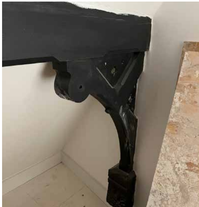
Image: Stone to external face, 'Union Club Company Limited.' Image: Roof timbers, visible at top floor level.
