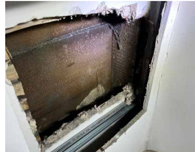
Image: Sarking to the underside of the tiled roof.
