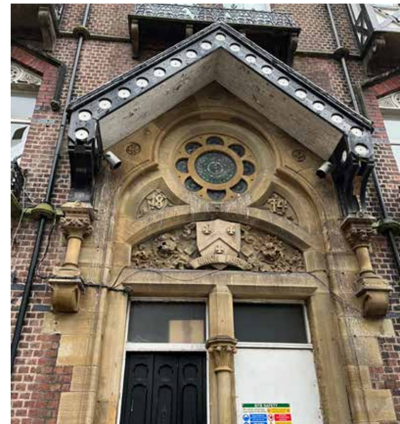
Image: Side elevation of Union Buildings. Image: Detail of entrance with date stone, Union Club 1874.
