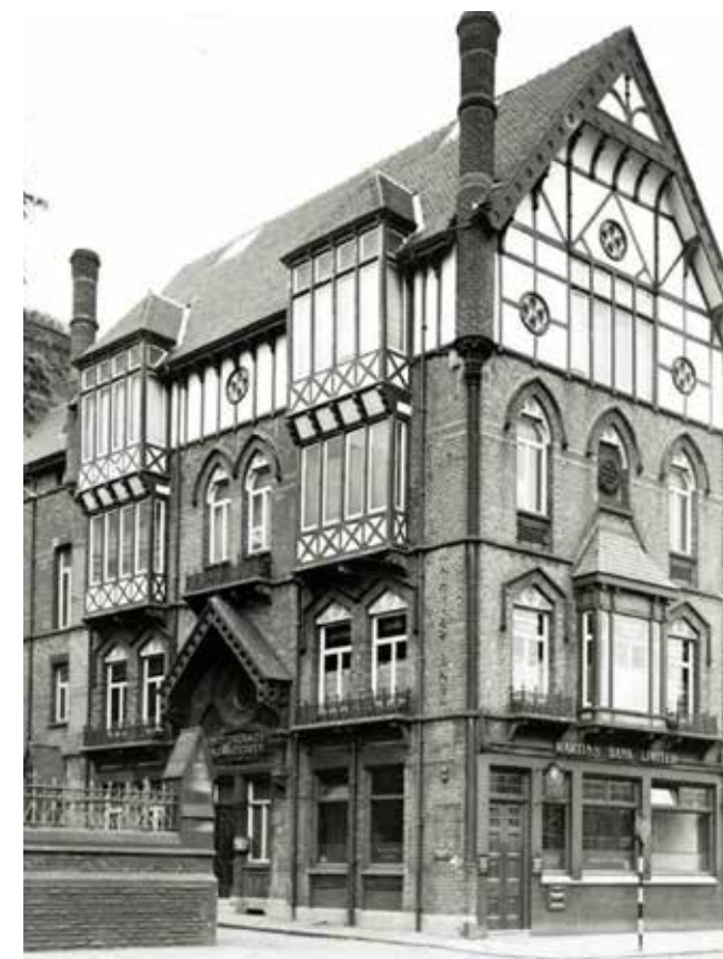
Image: Later half of 20th century. Outside plaster and window frames have been painted and roof re-tiled. Rooflight still visible.
