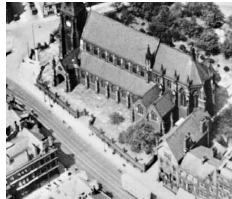
Image: Aerial view, 1927
