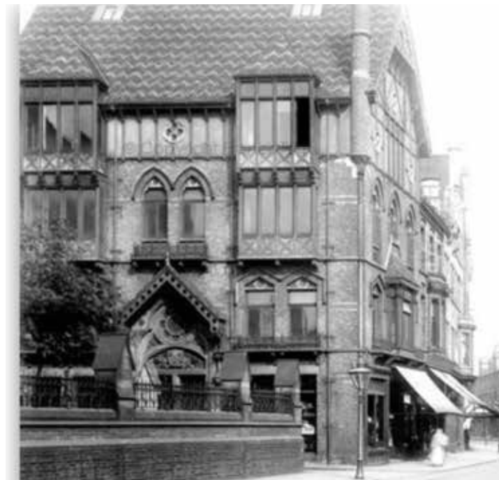
Image: Late 19th century– note roof lights zig zag tiling pattern and colour scheme of facade and window frames.
