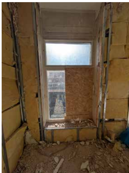
Images, Above: Example of windows to The Rock elevation. Below: Non-original example of window to The Rock elevation.
