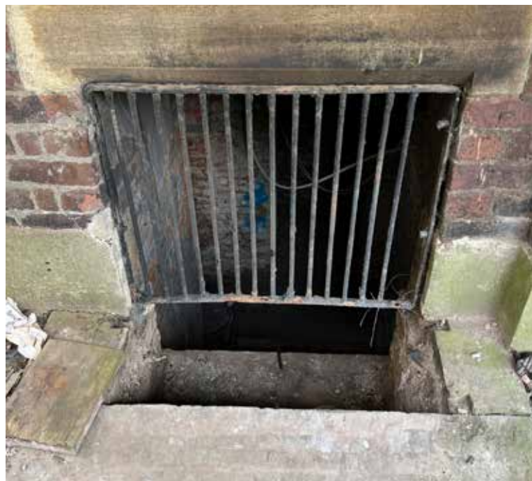
Images, Above: Basement showing existing openings. Below: Existing basement openings and pavement lightwell.
