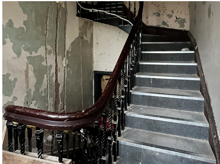
Image: Original staircase at top level.
