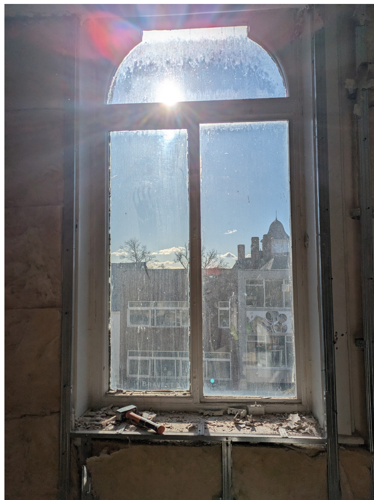
Image: Internal elevation of existing window.
