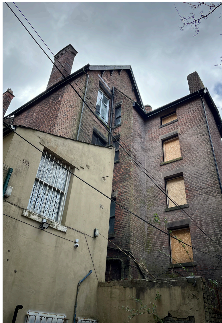
Image: Rear elevational view of the building.
