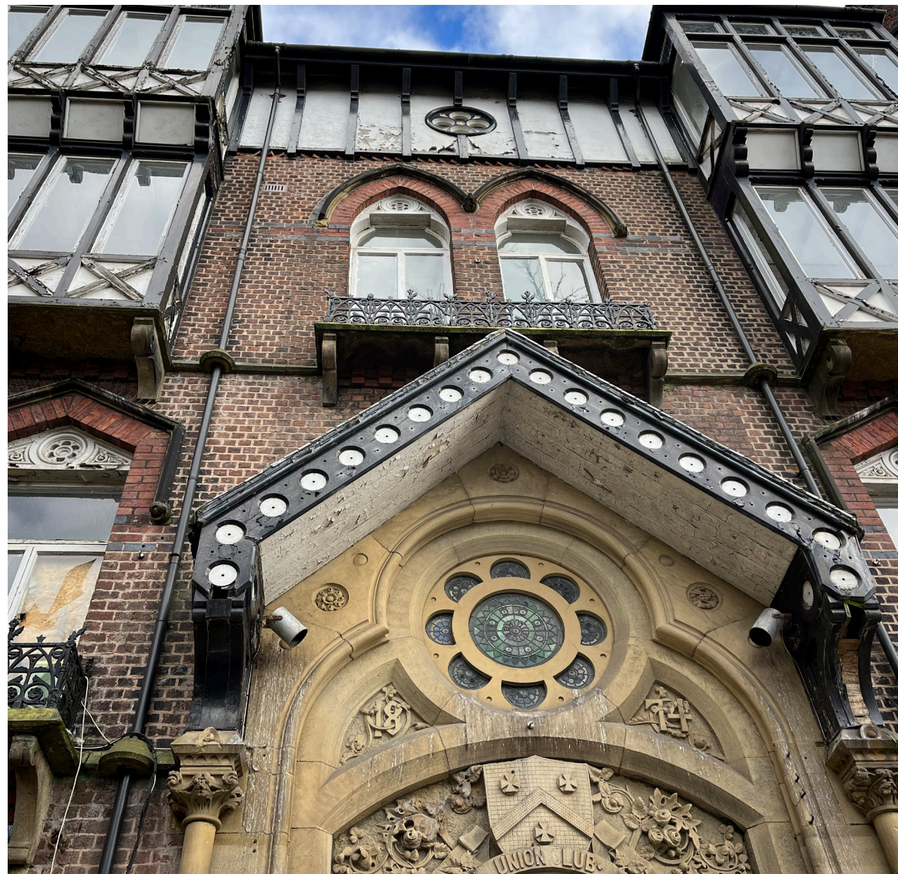
Image: External elevation showing main entrance.
