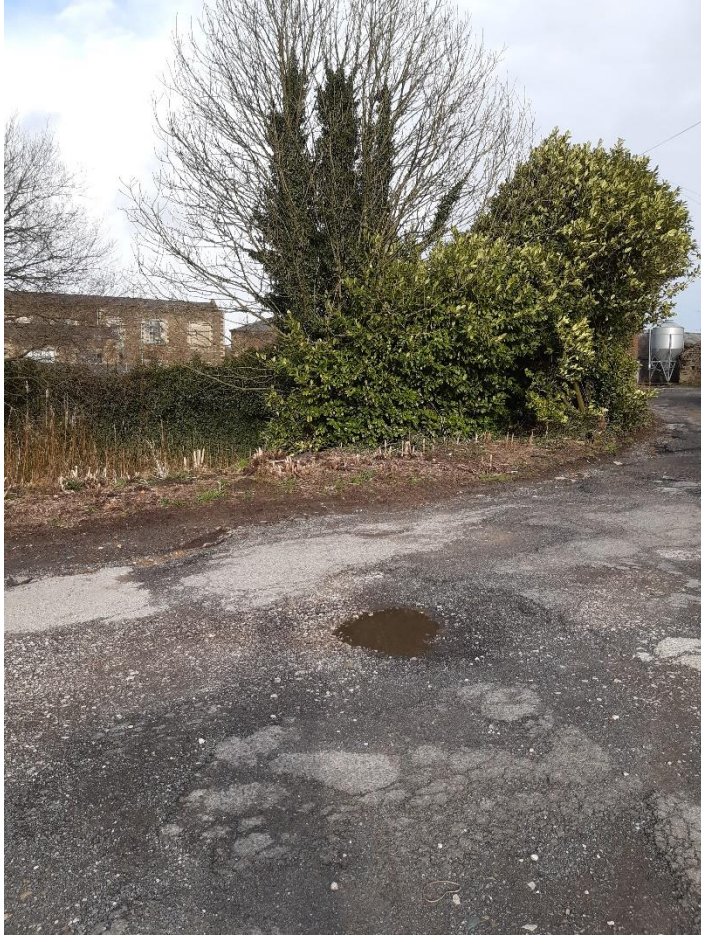
Pic 3 – JK area view to farm entrance
