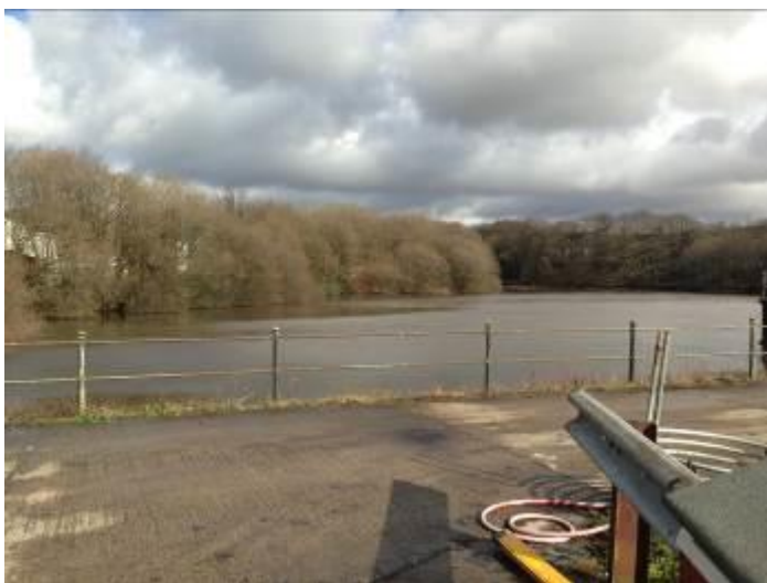
Plate 6 – Reservoir Looking North
