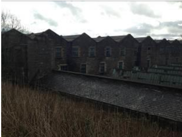
Plate 7 – Dam Looking Southeast Showing Split Level Site
