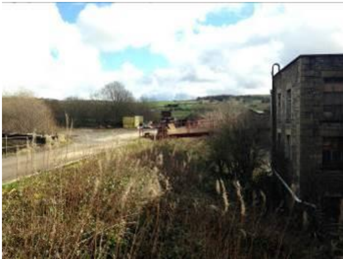
Plate 5 – Reservoir Dam Looking East
