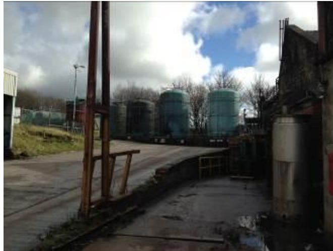
Plate 15 – Wider View of Tank farm to North
