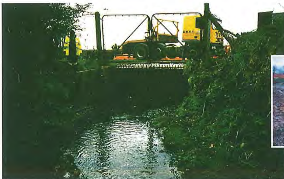
View of headscreen prior to removal
