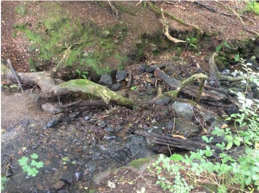
Figure 3-4: Large woody debris supplied into the channel with bank erosion
