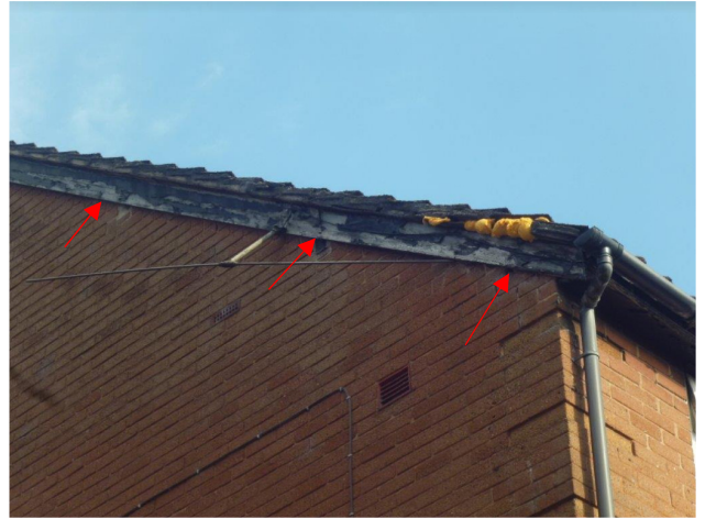
Facia board and repaired gaps in roof tiles along the northern elevation of the middle building.
