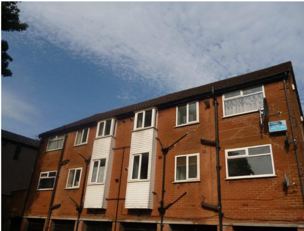
Western elevation of the most northern building. All three buildings of similar construction and layout.
