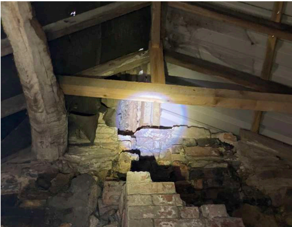
Inside the existing cottage
