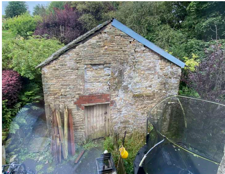
View from the main house at 1st floor level towards the cottage
