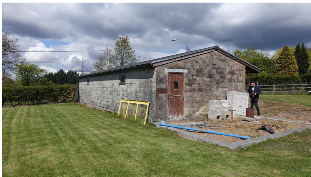
Existing stables with footings shown
