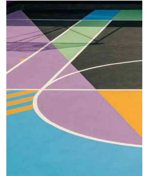
Basketball Shoot Court Porous asphalt with acrylic overlay artwork & thermoplastic lining
