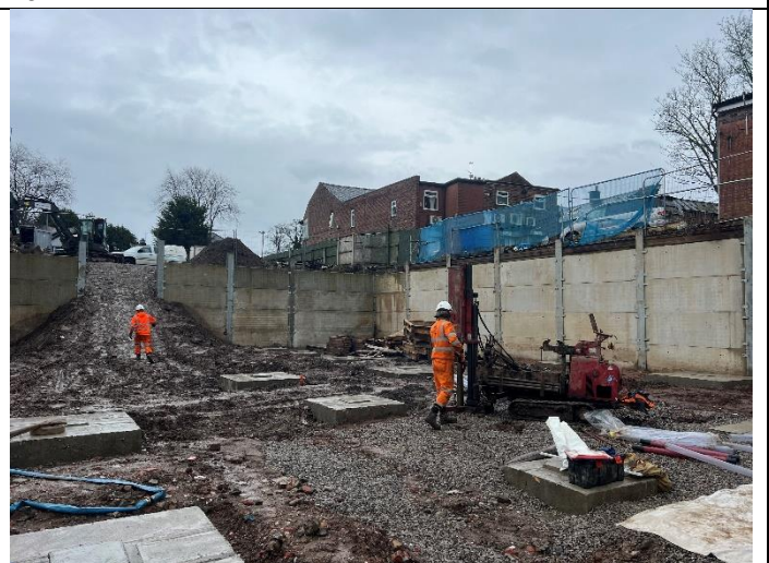
12: MW3 in progress
