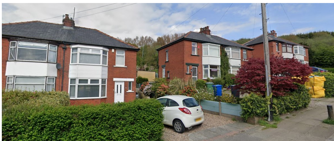
89 to 99 Bury New Road
