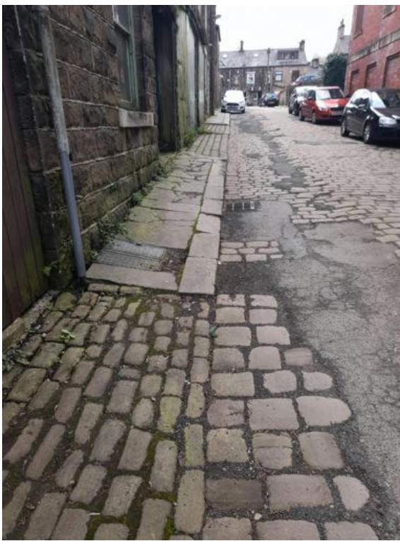
View 1 existing pavement
