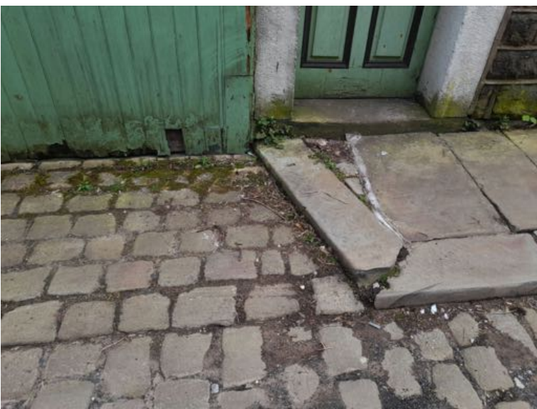
View 4 detail existing pavement
