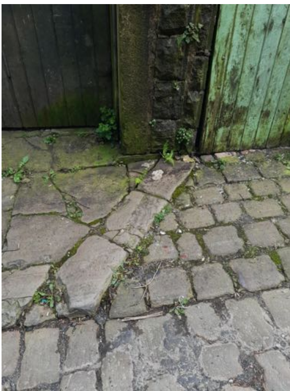
View 3 detail existing pavement
