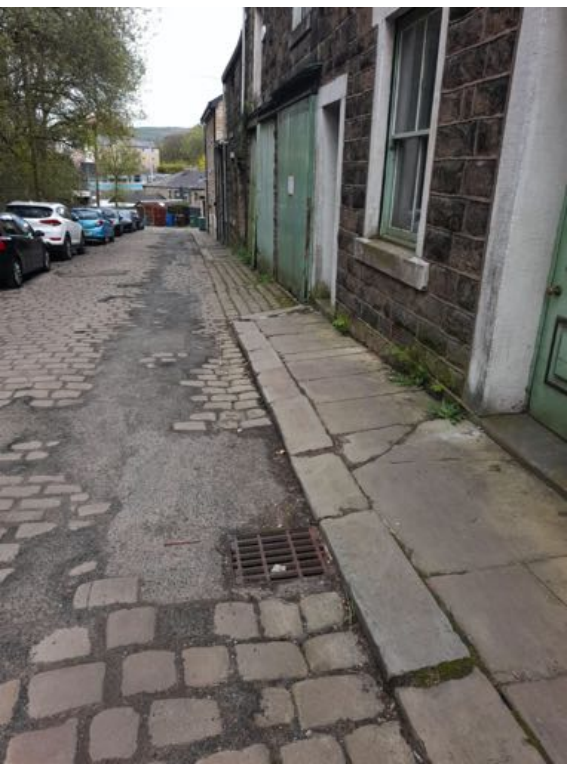
View 2 existing pavement
