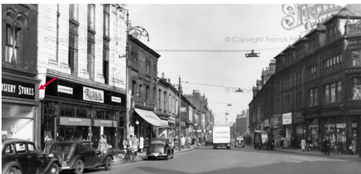
Figure 3.5 c.1950 view along The Rock, with a partial view of the shop front shown with an arrow (Francis Firth).
