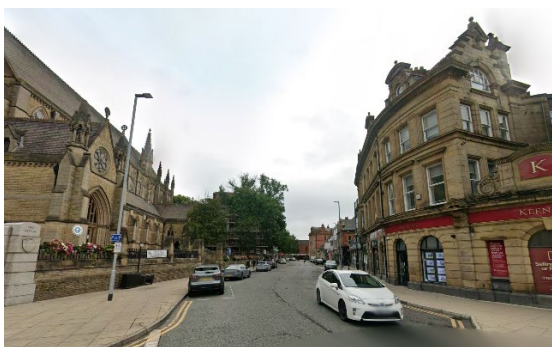
Figure 5.1 Key View east along The Rock (Google Street View)
