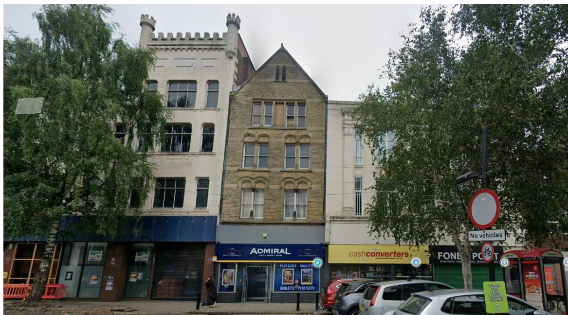
Figure 5.3 11-13 The Rock is included on the Council's draft local list and is identified as an 'unlisted building of merit' in the Bury Town Centre Conservation Area Appraisal (Google Street View).
