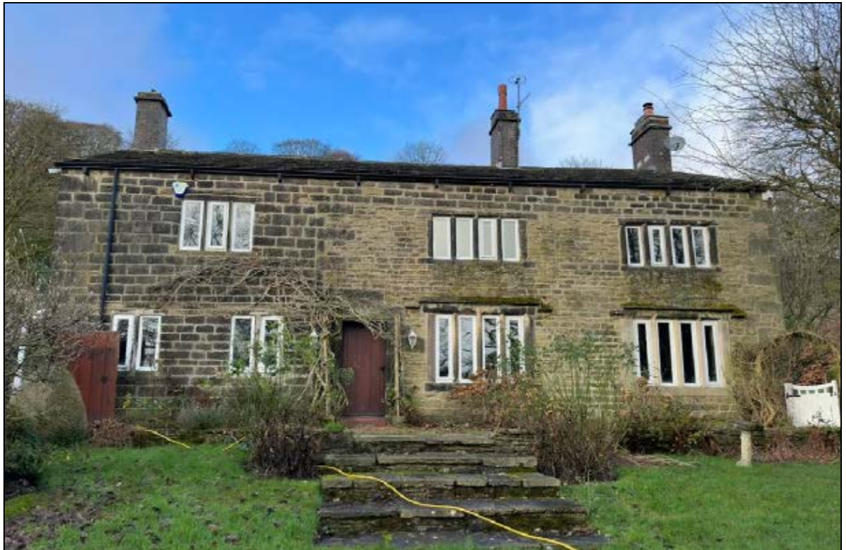
1. Front elevation of the listed building
