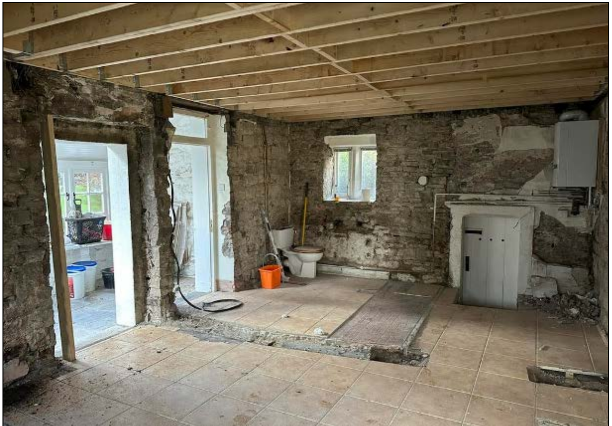
6. First bay, looking to rear and entrance to cellar
