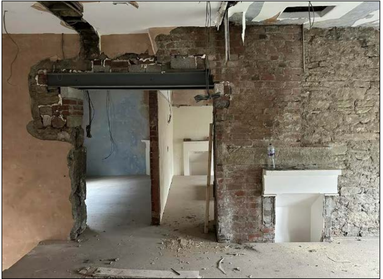
10. First floor view from second bay towards third bay, showing its division wall and fireplaces
