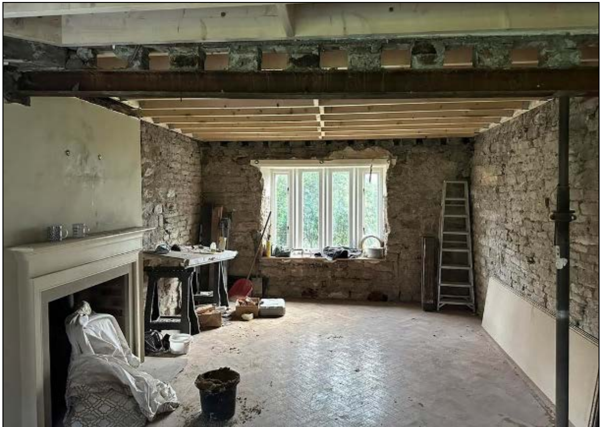
8. Third bay, showing non-original fireplace
