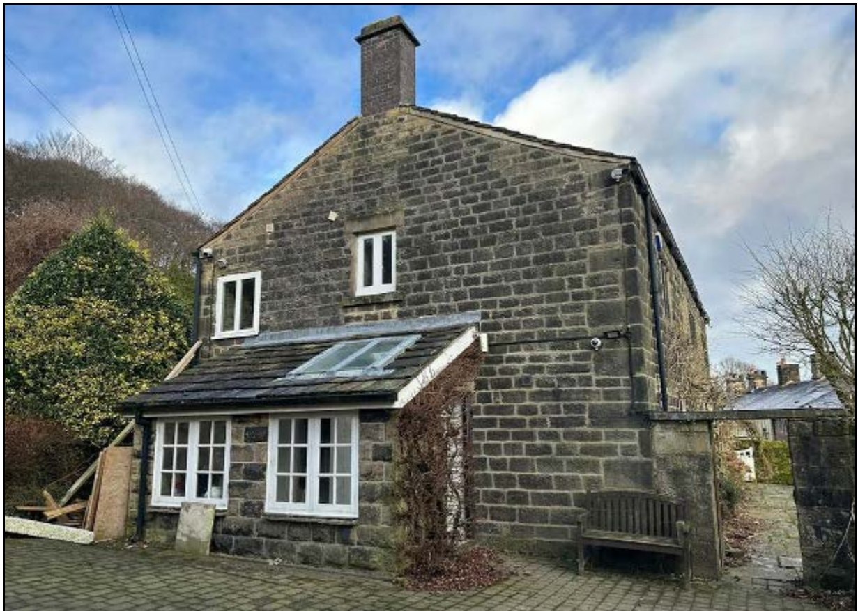
4. Lean-to on southwest elevation, probably 1980s
