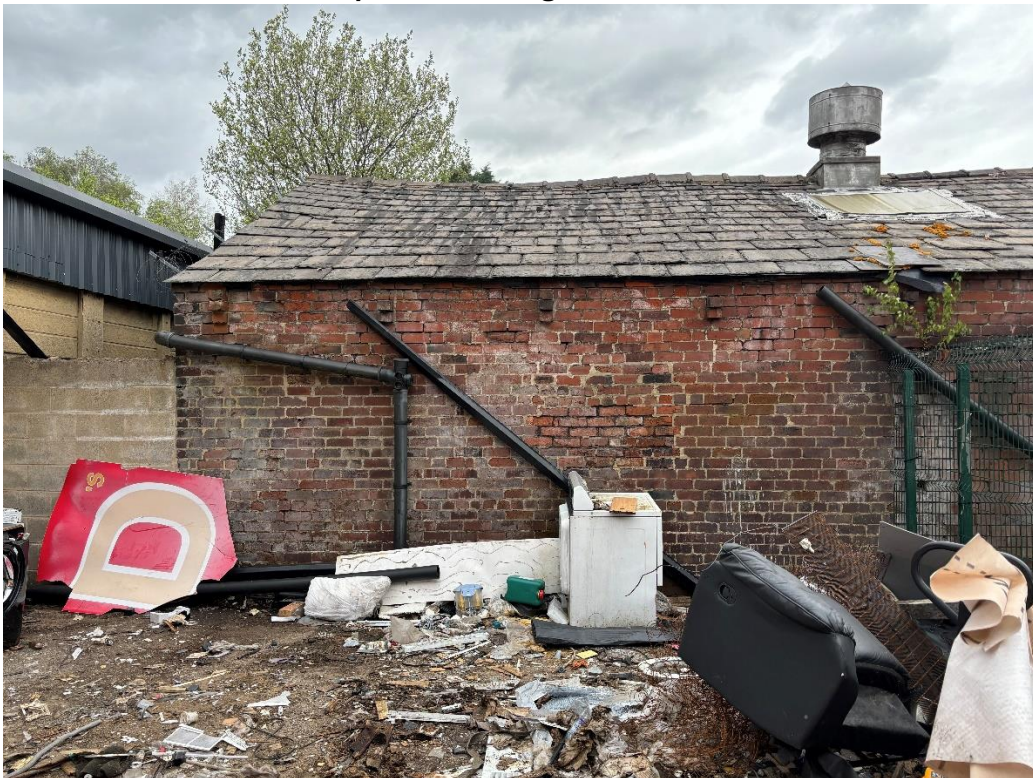
Southern elevation of rear part of building
