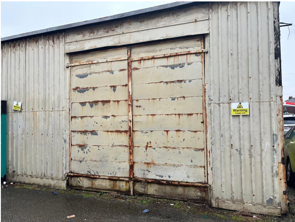
Access doors in Southern elevation
