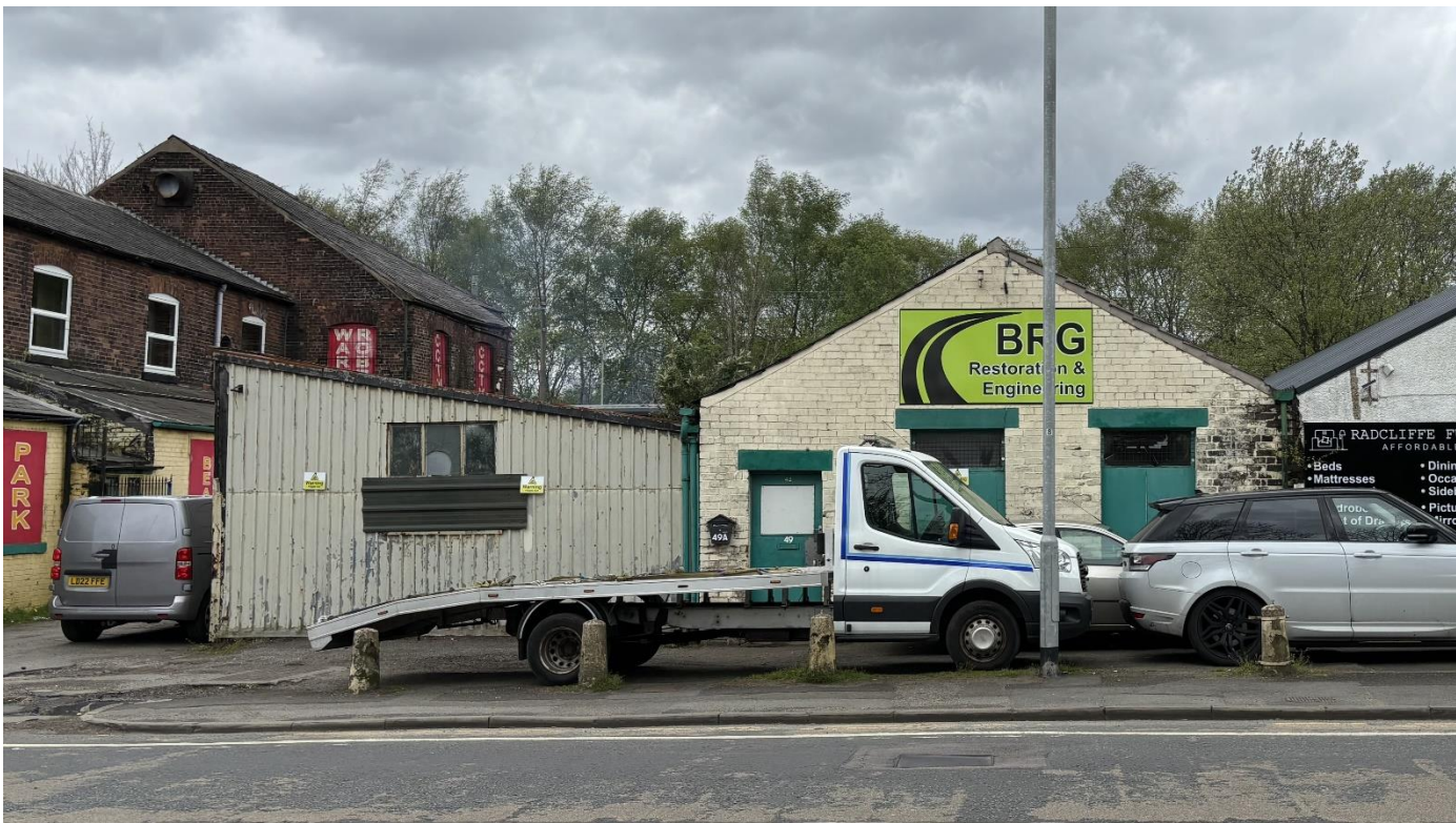
Front elevation showing Bury Road works (47) behind
