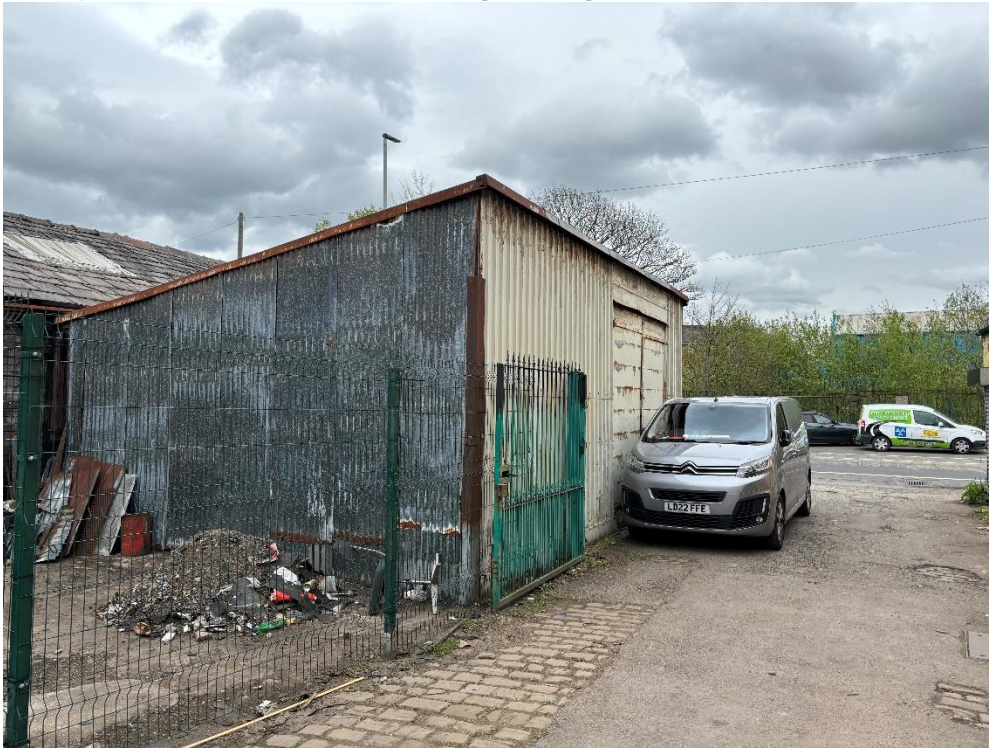
Monopitch side extension to building looking towards Bury Road
