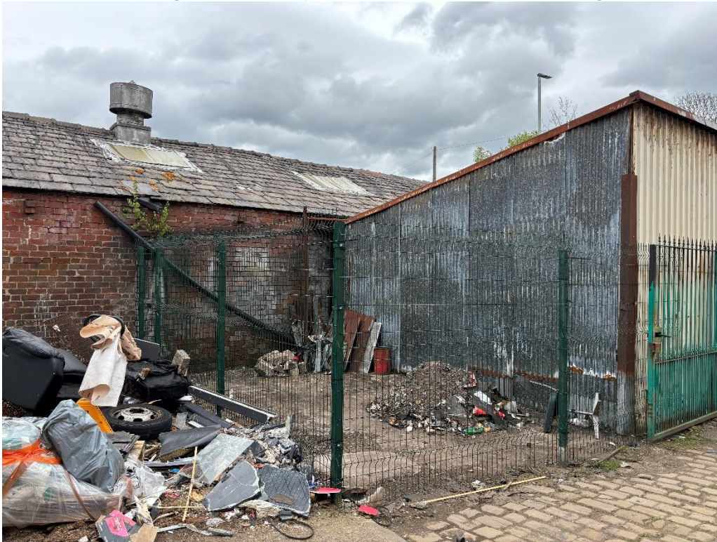
Fence demarcating site boundary and location of former building now demolished as unsafe
