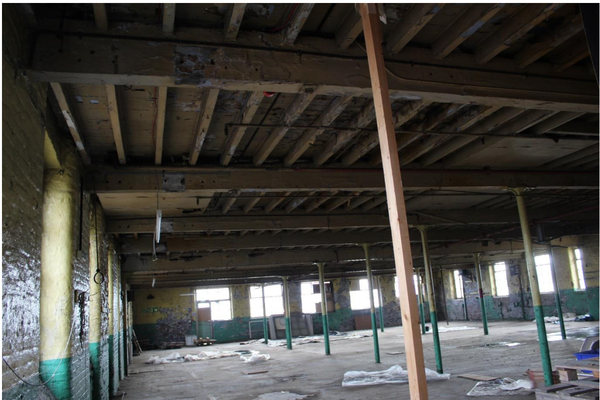
Plate 21 – 2 nd Floor Original Range
