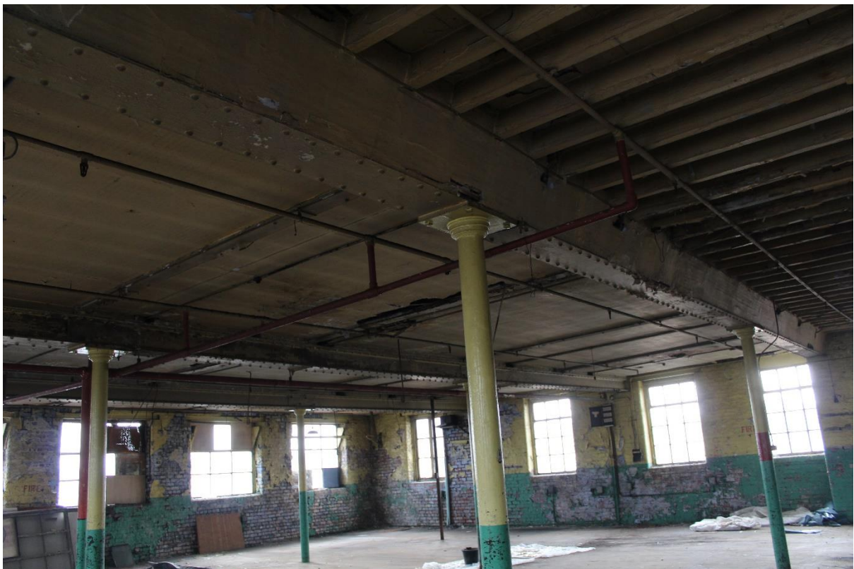
Plate 23 – 2 nd Floor Extension
