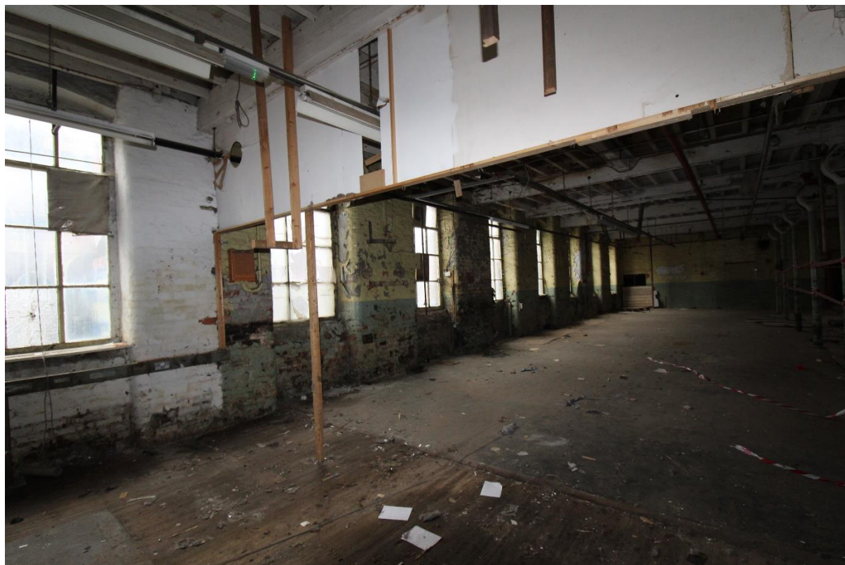
Plate 12 – Ground Floor Original Range
