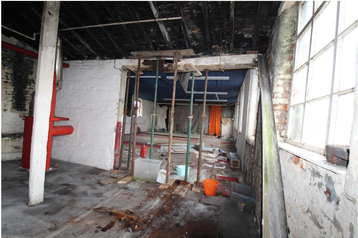
Plate 20 – 1 st Floor, Boiler House
