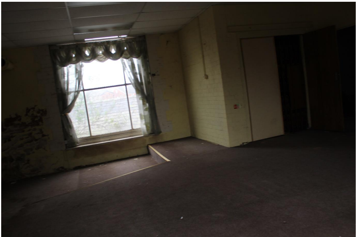
Plate 19 – 1 st Floor, Engine House
