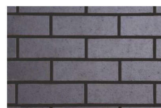
Brickwork - Staffordshire Blue Engineering Brick
