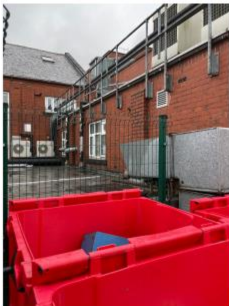
Accommodation above basement plant room, to be demolished
