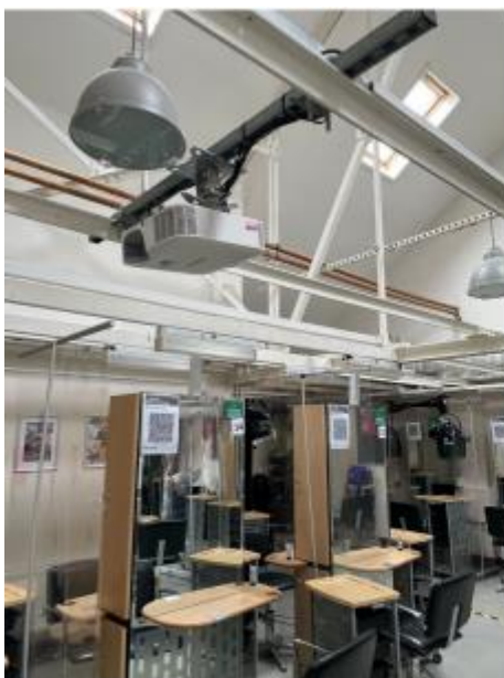
Interior view, exposed structure and services, poor light and views, low quality teaching space
