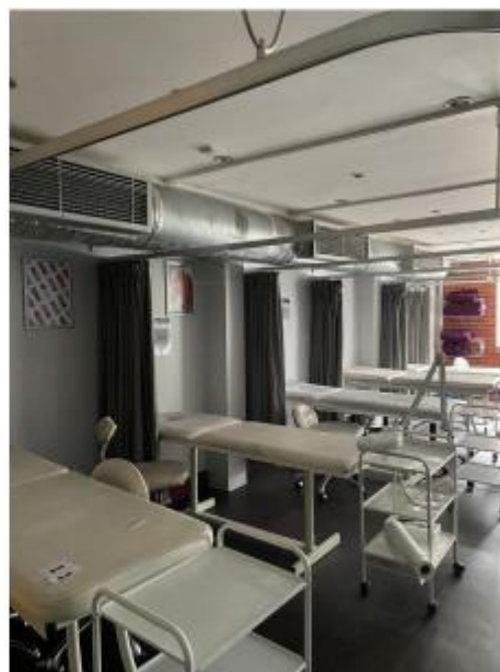
Internal view, low ceilings, lack of windows, exposed services, very low quality teaching space
