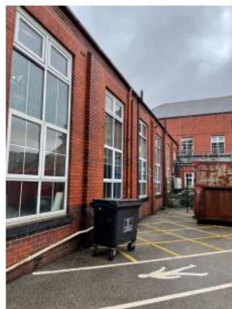
South elevation of building to be demolished
