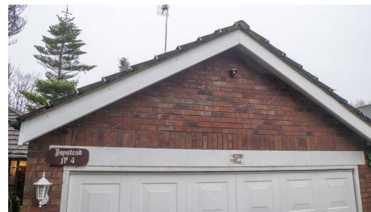
3. Garage on front of site adjacent to bungalow
