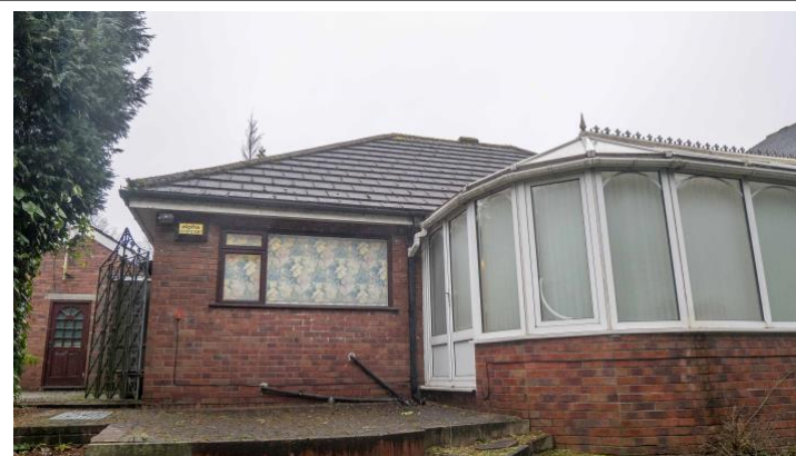
5. Roof and conservatory detail
