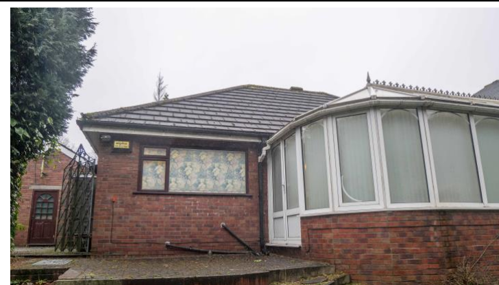
6. Rear elevation with conservatory
