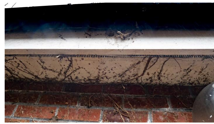
3. Ventilation for soffits
