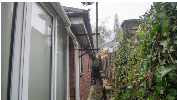
4. Side elevation, all extended soffit boxes in good condition
