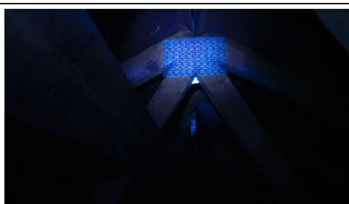
8. All areas inspected using UV lighting to identify any evidence of bat activity
