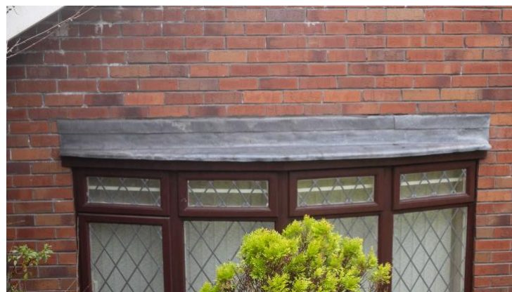
2. Deetail of flashing over front bay windows
