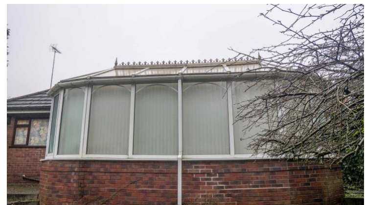
4. Rear elevation with conservatory
