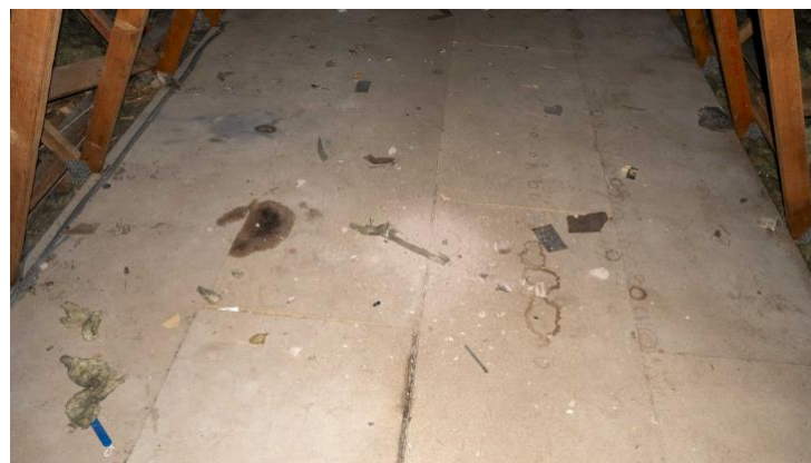
2. All areas of loft space floor boarded giving easy access
