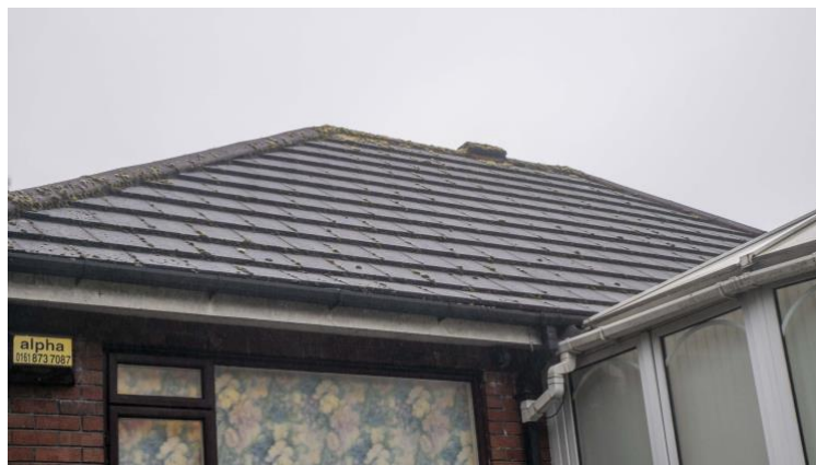
1. Ridge and roof tile detail rear elevation
