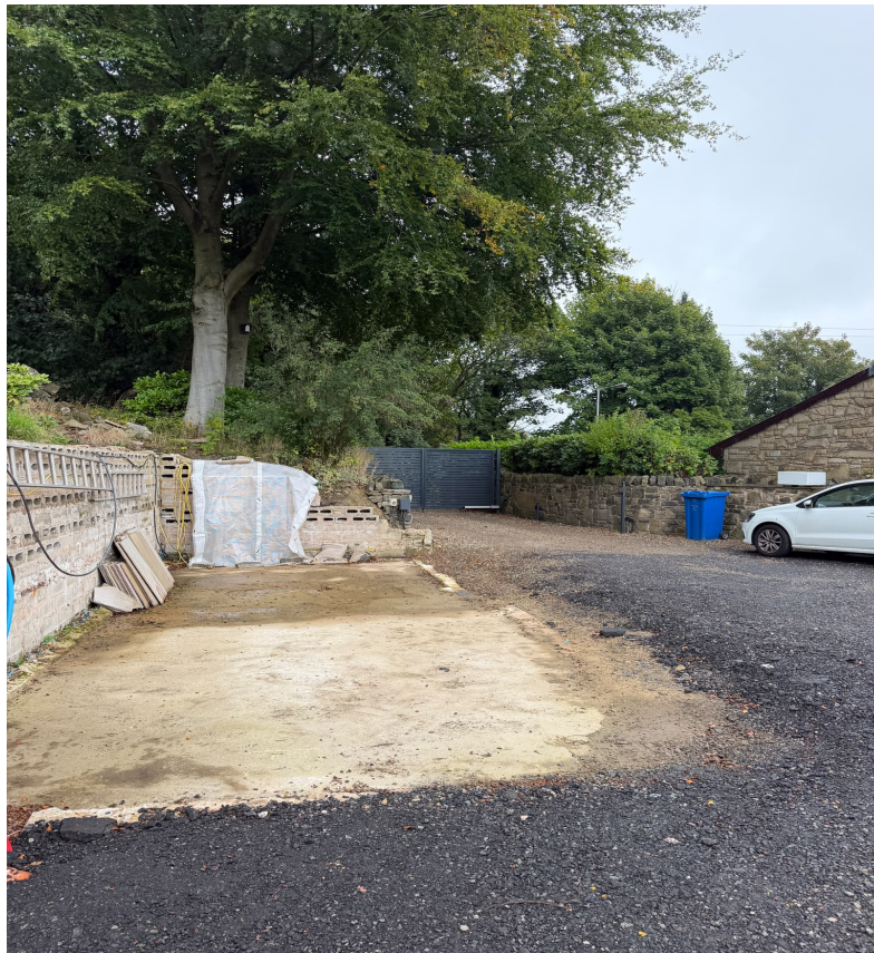
Image of site of Garage post demolition
