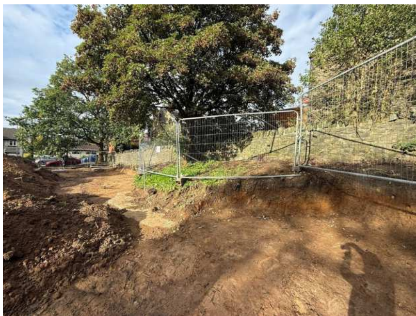
Photo 4: Wide view showing the retained Sycamore behind the protected area and the excavation face outside the fenced zone.
