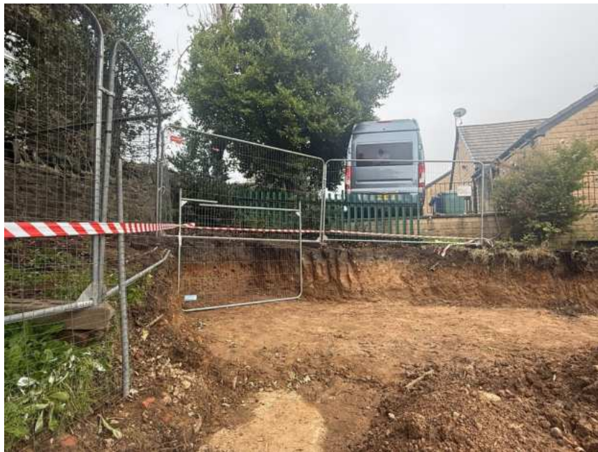
Photo 10: Further view of the excavated construction zone and retained tree-protection boundary.
