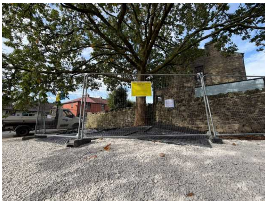
Photo 16: Completed protected area around T8 showing fencing / warning signage, ground-protection boards and permeable aggregate working surface.
