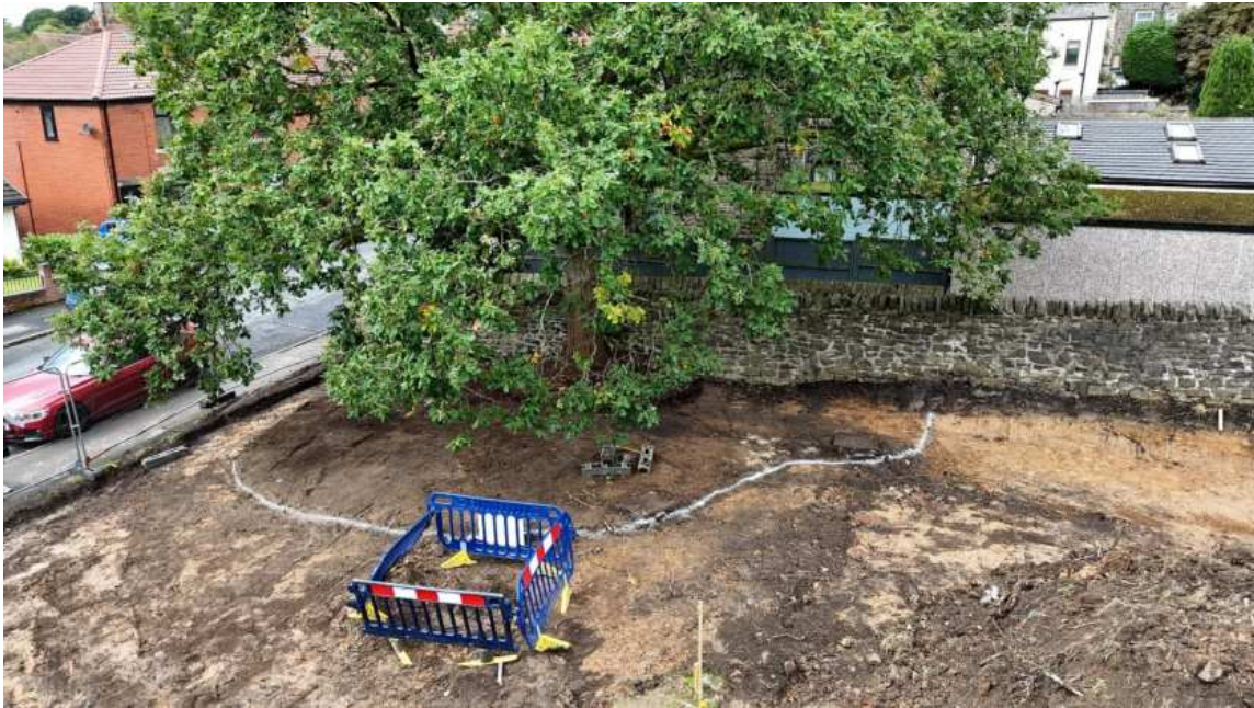
Photo 11: High-level view of T8 Pedunculate Oak with the RPA / working boundary marked on the prepared ground.
