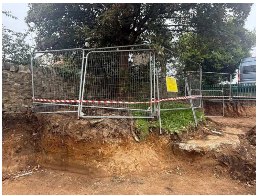
Photo 8: Retained Sycamore enclosed by temporary fencing with tree-protection warning signage visible.
