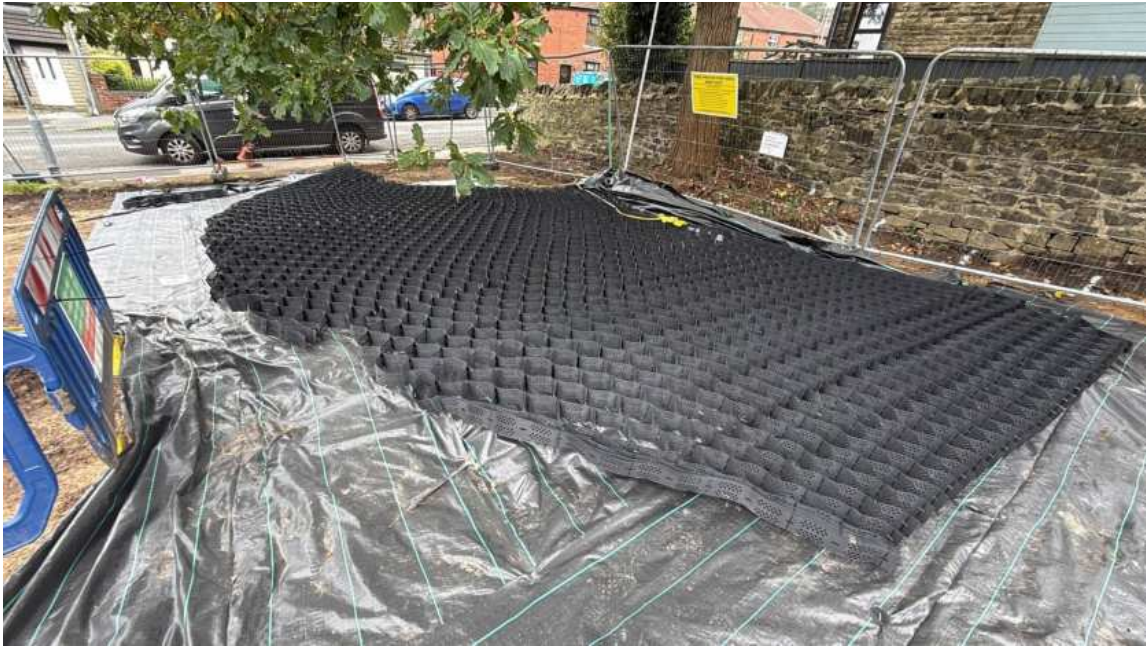
Photo 17: Base geotextile laid over the prepared formation with cellular confinement expanded across the defined area; tree-protection fencing remains in place.
