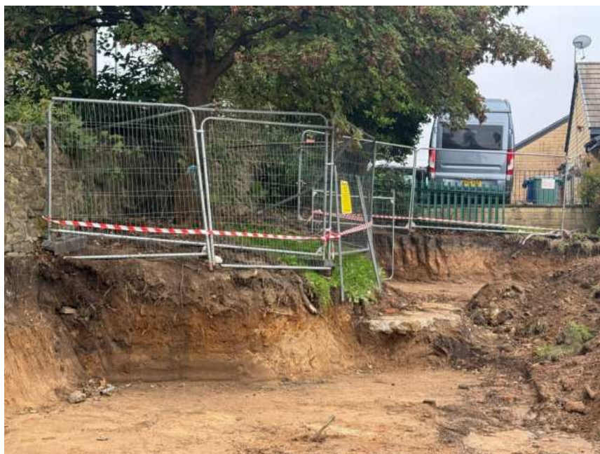
Photo 7: Retained Sycamore with protective fencing, warning tape and controlled access around the tree-protection area.
