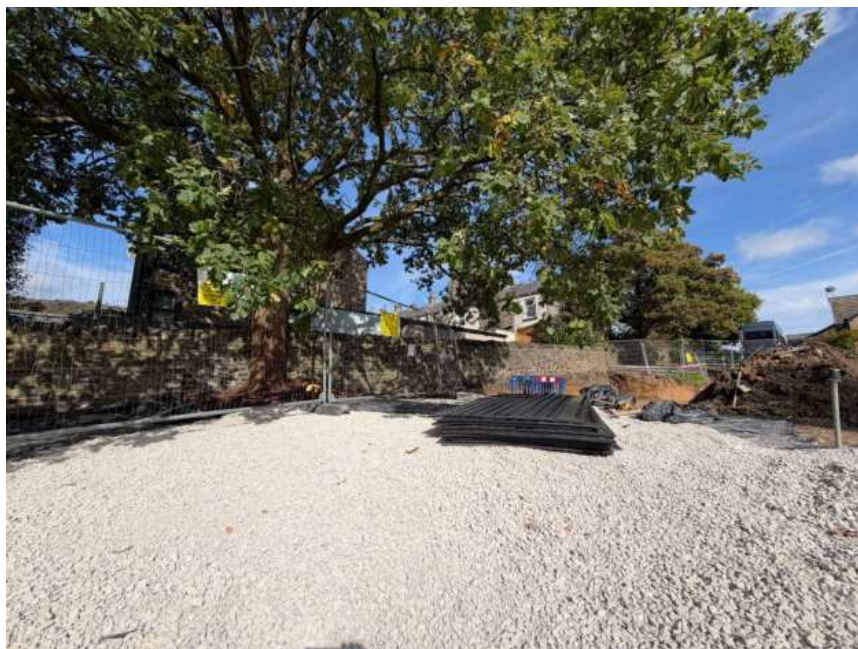
Photo 14: Open-graded aggregate working layer installed adjacent to T8, with protective fencing and warning signage maintained.
