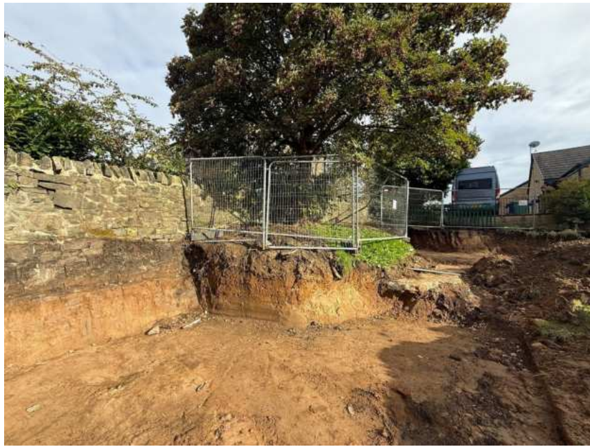
Photo 5: Excavation geometry around the retained tree area, with temporary fencing positioned along the upper edge of the protected zone.
