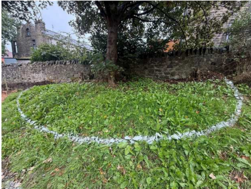
Photo 1: Initial view of the retained Sycamore and the marked protection / working boundary prior to the later excavation sequence.
