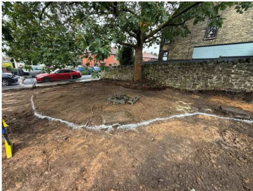
Photo 12: Ground-level view of the marked RPA / construction interface around T8 Oak.
