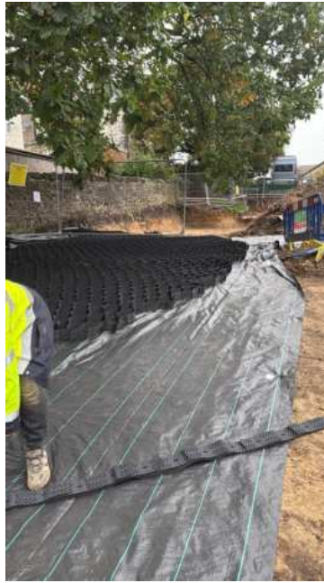
Photo 19: Installation-stage view showing geotextile beneath the expanded confinement cells before aggregate infill.
