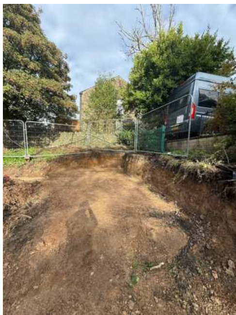
Photo 3: Excavated construction area adjacent to retained tree protection zone; temporary fencing separates the tree area from the excavation.
