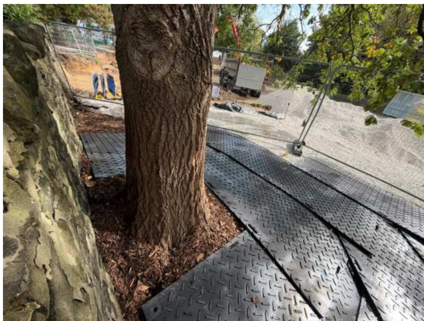
Photo 15: Interlinked ground-protection boards positioned around the Oak stem with aggregate working layer beyond.
