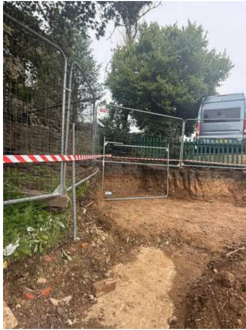
Photo 9: Controlled route / working area adjacent to the retained tree zone with temporary fencing maintained.
