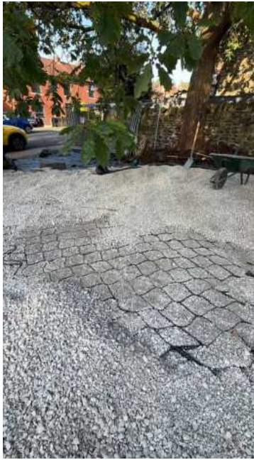
Photo 21: Filled cellular confinement adjacent to T8 Oak, with open-graded aggregate placed through and over the cell matrix.
