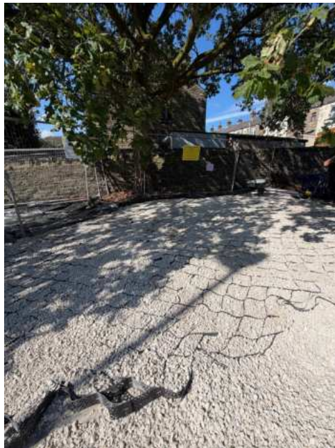
Photo 18: Cellular confinement system substantially filled with open-graded aggregate, with confinement matrix visible at the surface.
