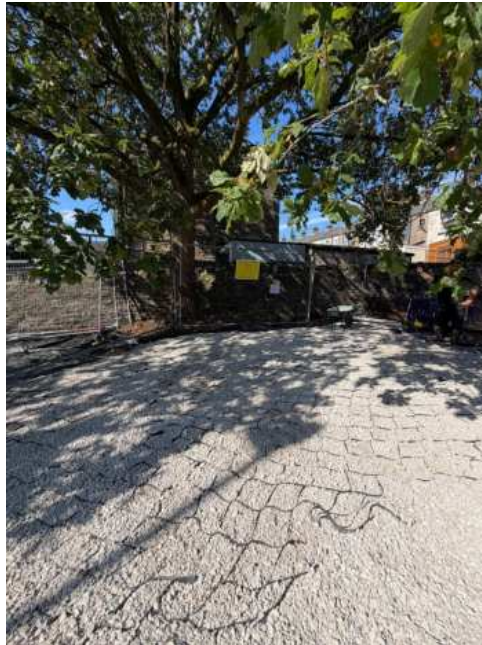
Photo 22: General completed installation view showing the cellular matrix visible within the aggregate surface beneath the Oak canopy.
