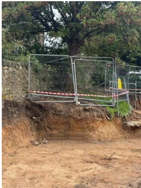
Photo 6: Closer view of the Sycamore and temporary protective fencing above the excavation face.
