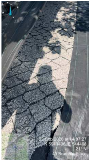
Photo 20: Timestamped close view showing the cellular confinement matrix filled with open-graded aggregate.
