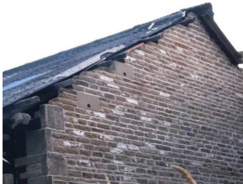
Example of Forticrete boxes in situ
