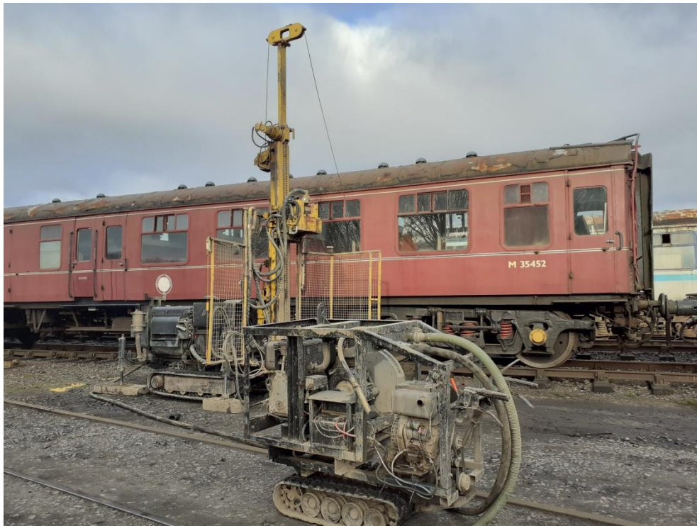
Borehole TDS 2 View west
