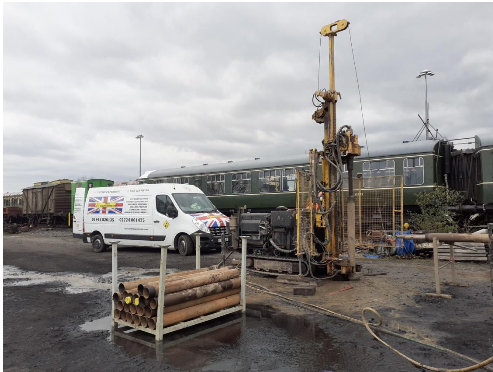
Borehole TDS 1B View south-south west
