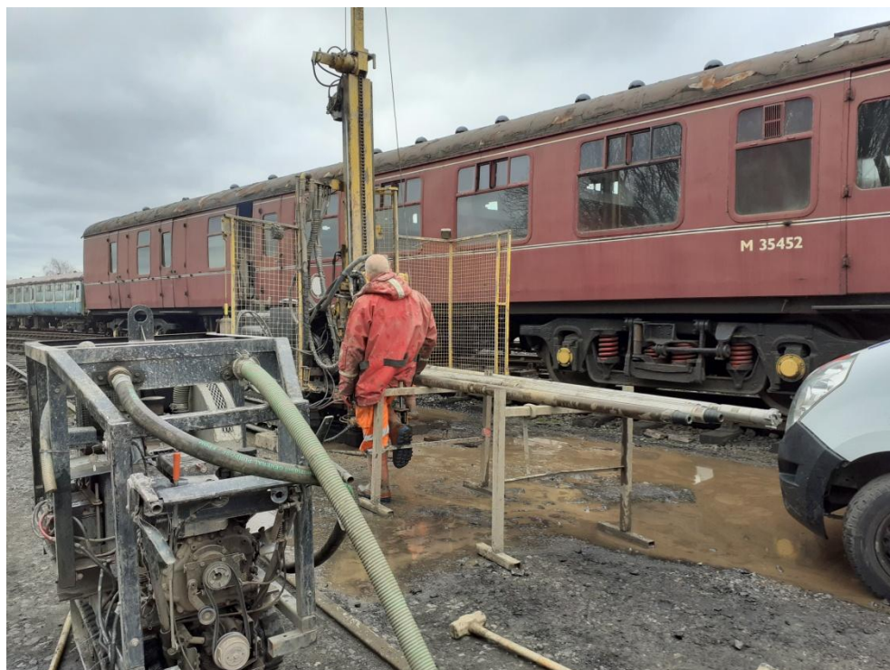
Borehole TDS 2 View south west
