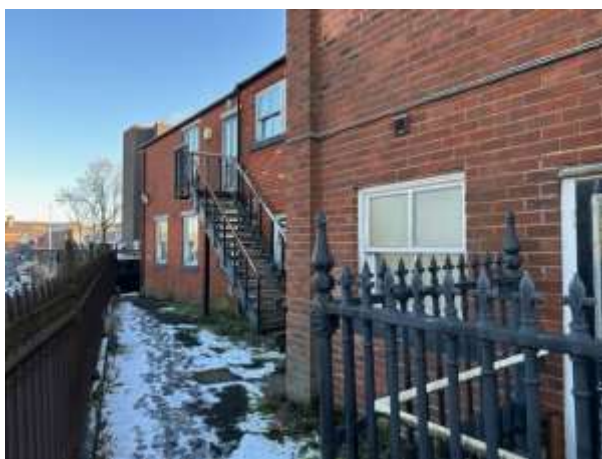
Image 02 – Gable elevation (apartment 1) Existing brick facings
