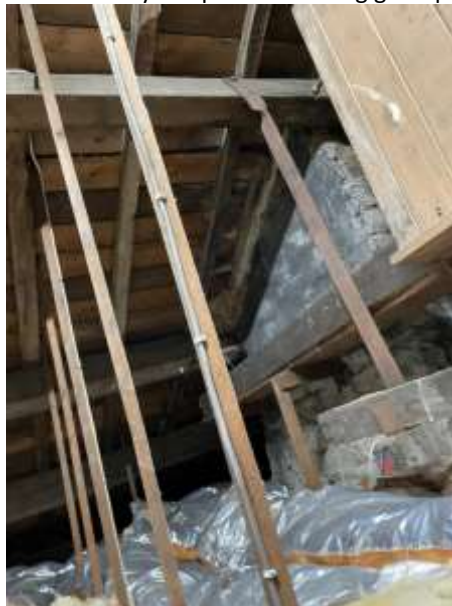
Roof structure includes traditional timber purlins and rafters, supported locally timber truss framing.
