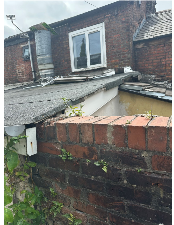
Currently the site is disused and in need of repair
