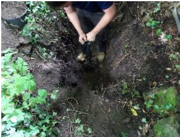
Trail pit 1 – excavation to 1.3m
