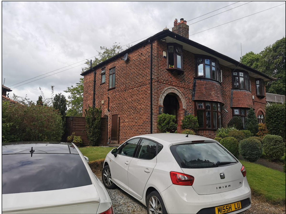
Site Photo (View C)
