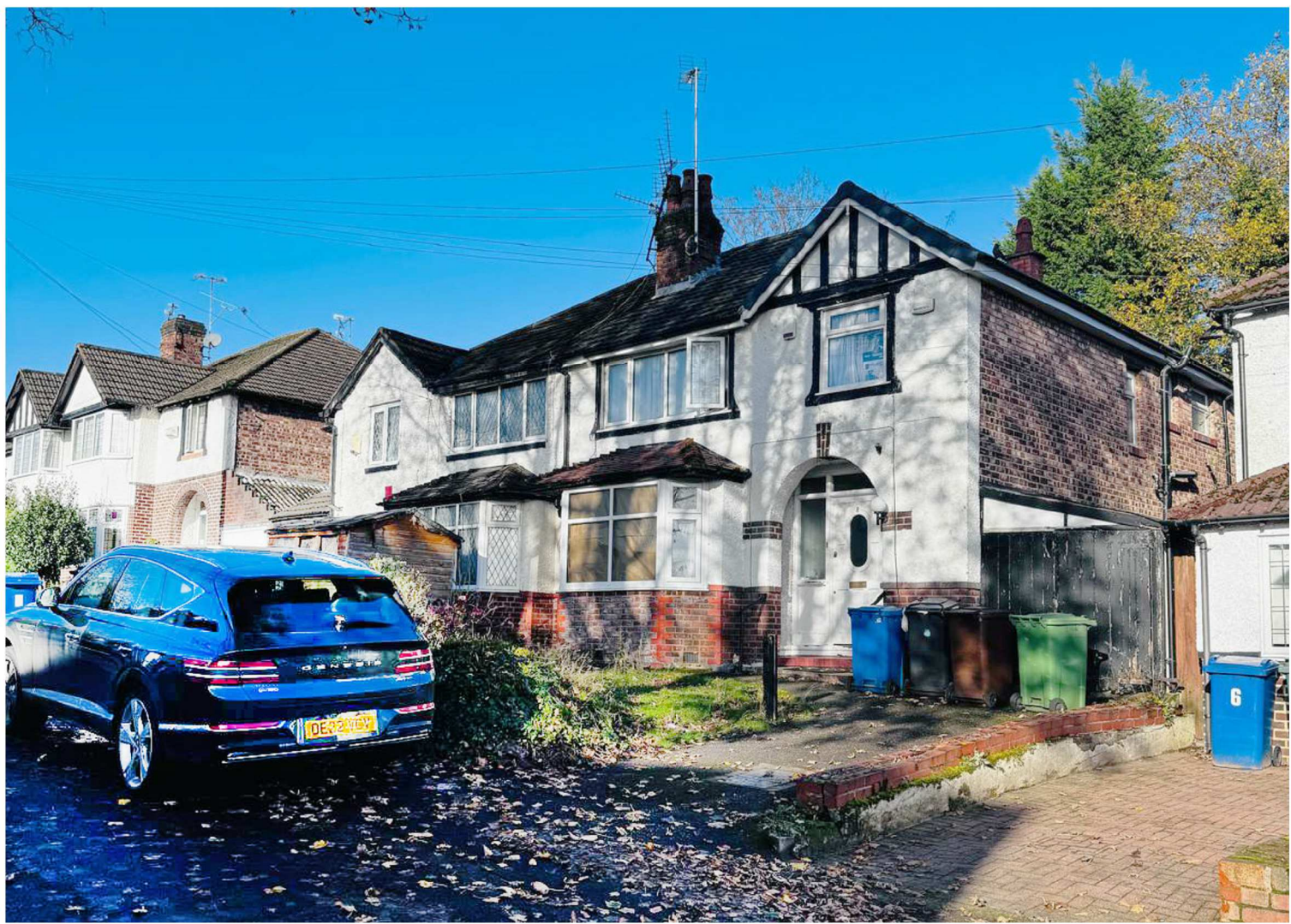
Existing Street Scene Photograph
