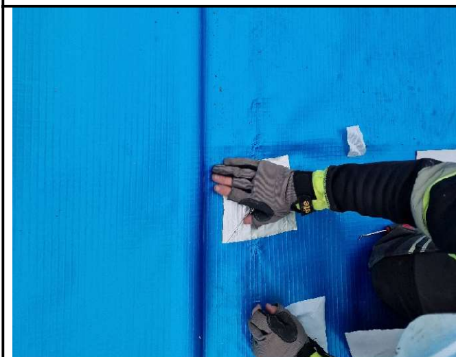
Figure 11 -- Area in Fig 10 over patched with Visqueen Pro Detail tape
