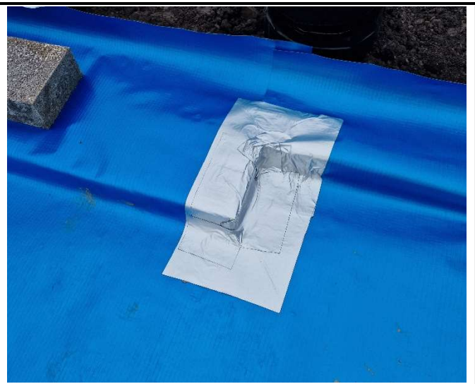
Figure 8 -- Corners detailed with Visqueen PRO Detail Tape
