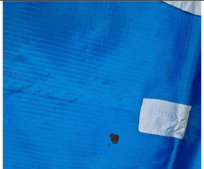
Figure 6 – Sheet sealed by hand held heat welding
