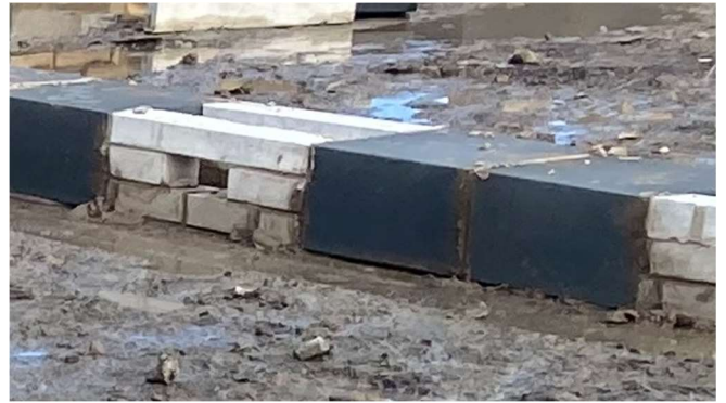
Figure 2 – Through vent and depth of trench block is depth of void, once beams are placed.
