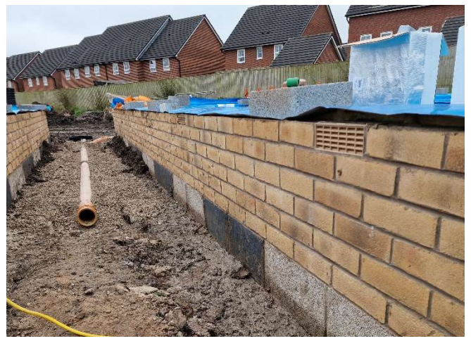
Figure 4 – Perimeter Sub floor vents in place
