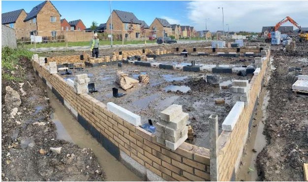
Figure 1 -- General View Across Plot 51/52 during subfloor construction note Perimeter and through vents
