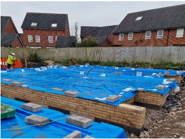
Figure 3 – Plot 51/52 with membrane in place
