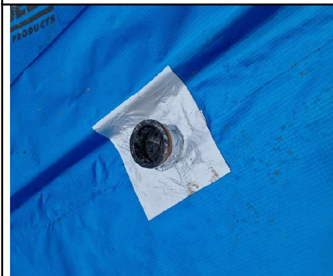
Figure 9 -- Service penetrations detailed well
