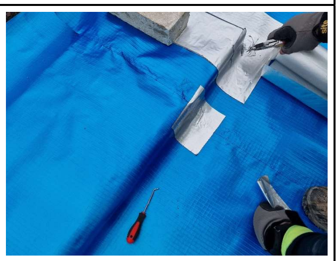
Figure 18 weak seam strengthened with visqueen pro detail tape
