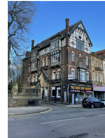
Street view showing facade
